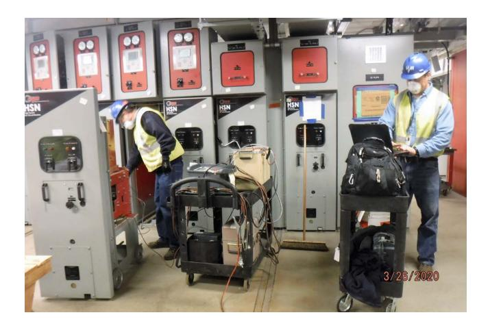
The picture above depicts the CS084 contractor performing tests on various feeder breakers in the C08 substation in Queens for the East Side Access Project. This month's procurement package includes a procurement action for the CS084 Contract.
