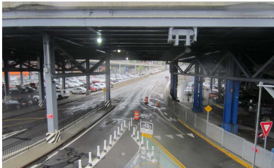
Existing crew facilities
