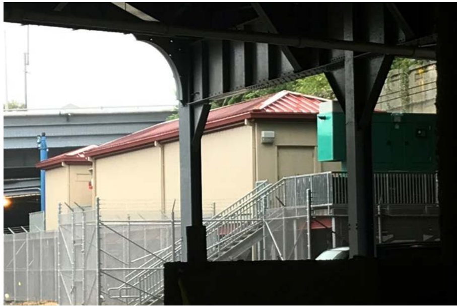
Raised SIR Signal House
