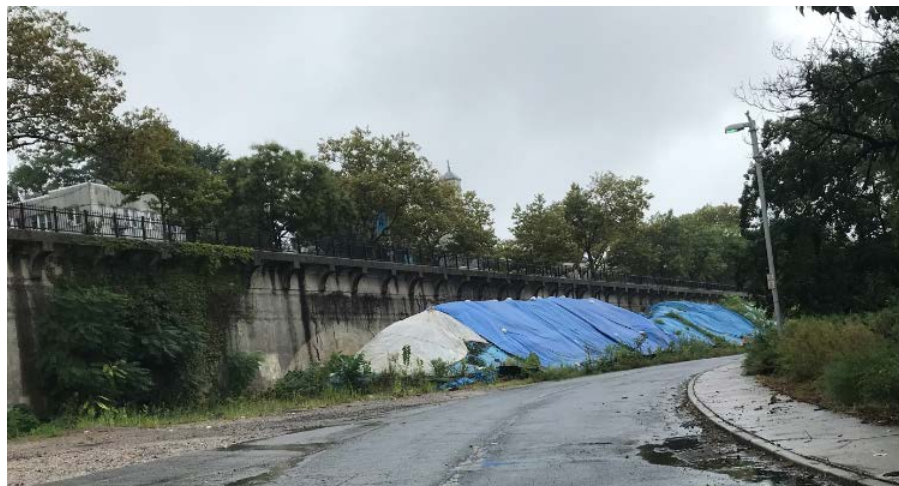
Existing spoils along Bank Street
