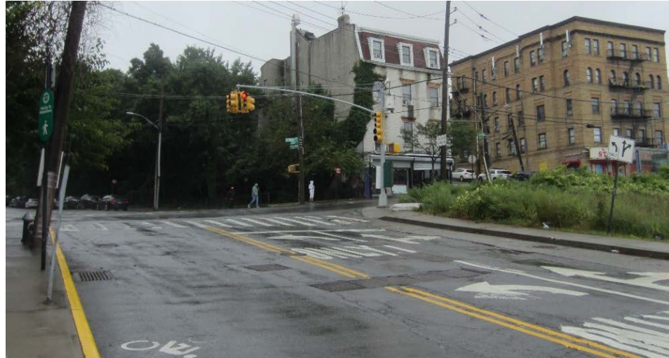
Existing Nicholas Street intersection with Richmond Terrace and NY Wheel Garage
