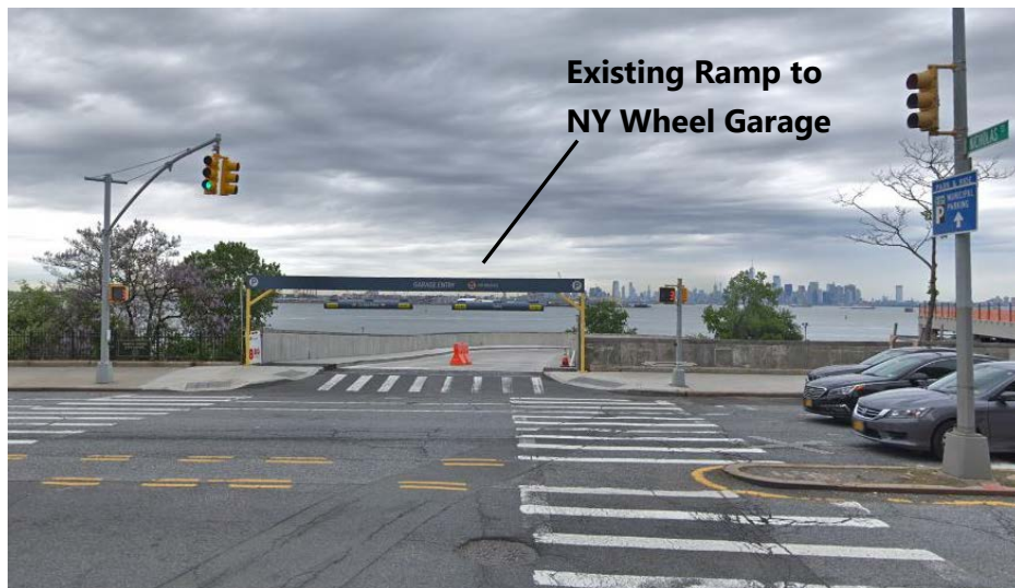
Existing Nicholas Street intersection with Richmond Terrace and NY Wheel Garage. The proposed BRT ramp would be located to the left of the existing garage ramp.
