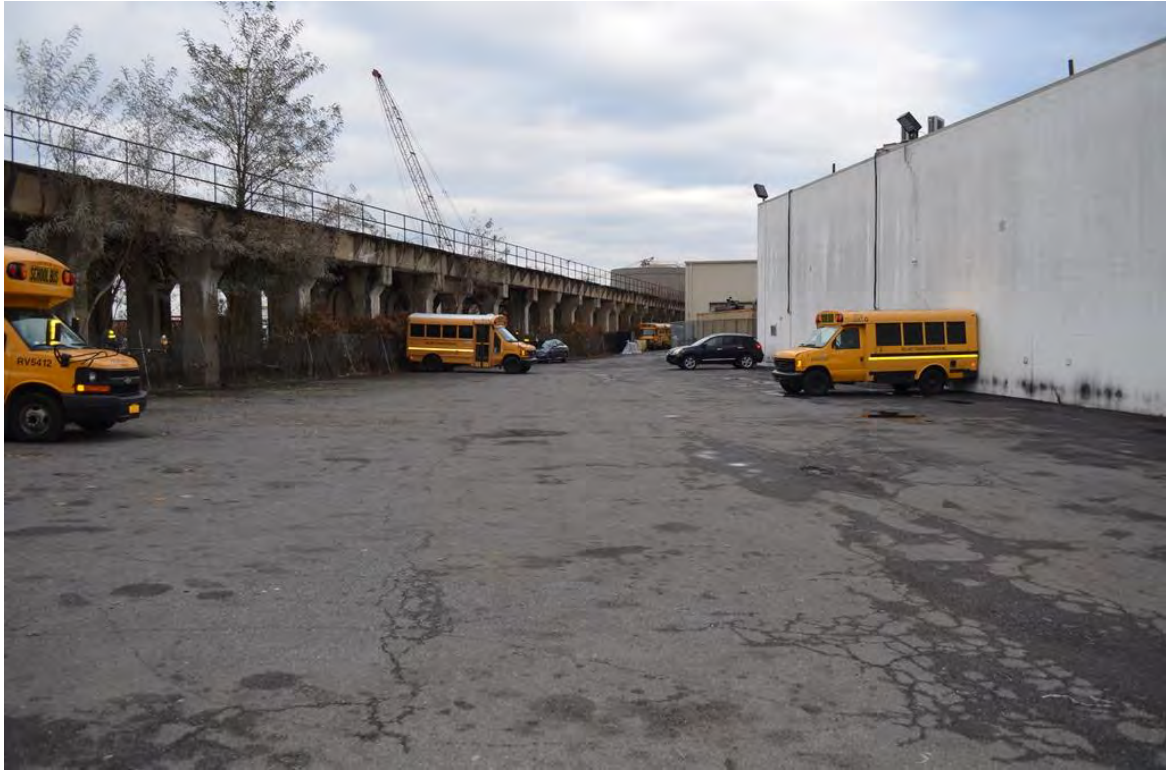
Photograph R.13. Section 4, detail of the viaduct near Richmond Terrace. View looking northeast.
