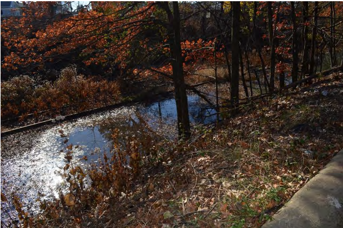
Photograph R.20. Section 5, the open cut filled with water near Winant Street. View looking southwest.
