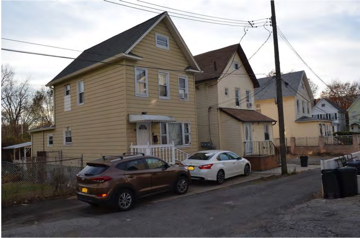
Photograph 6.18. Lockman Place north of the ROW. From left: 4, 3 and 1 Lockman Place (Block 1236, Lots 124, 125, and 127). View looking southwest.
