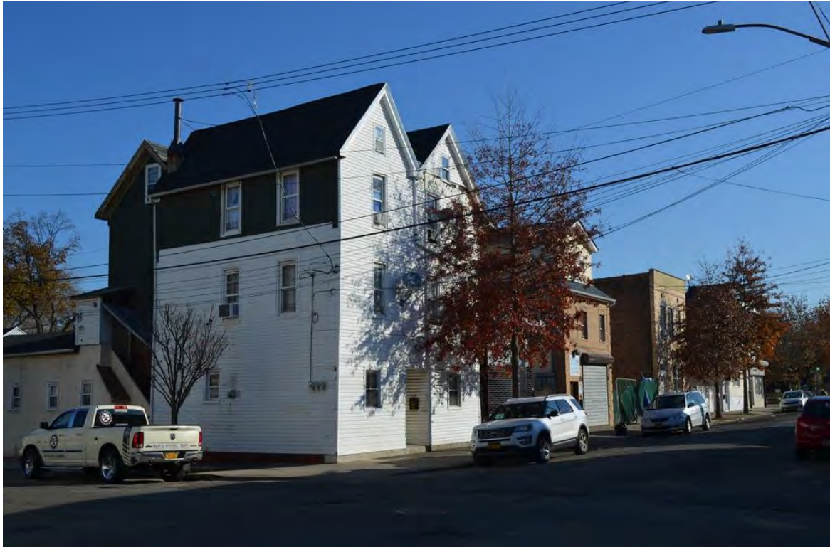
Photograph 4.23. Grove Avenue between Faber Street and Maple Avenue. At left is 59 Grove Avenue (Block 1074, Lot 9). View looking northeast.
