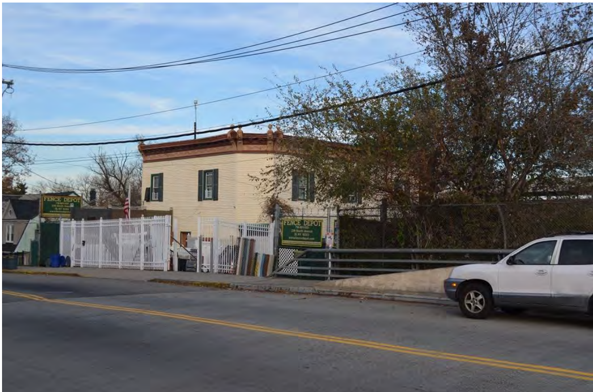
Photograph 6.11. South Avenue at the edge of the overpass north of the ROW. 237 South Avenue (Block 1257, Lot 9). View looking northeast.
