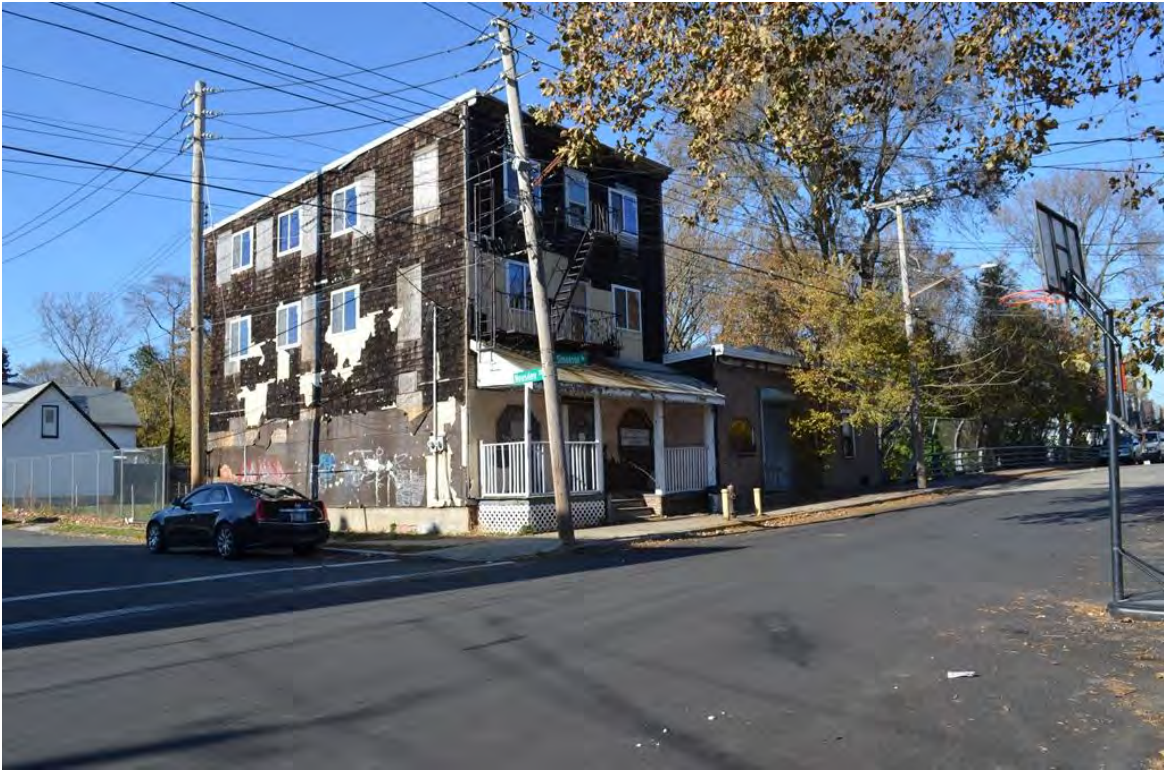
Photograph 5.28. Simonson Avenue south of the overpass. 126 Simonson Avenue (Block 1186, Lot 124). View looking northwest.
