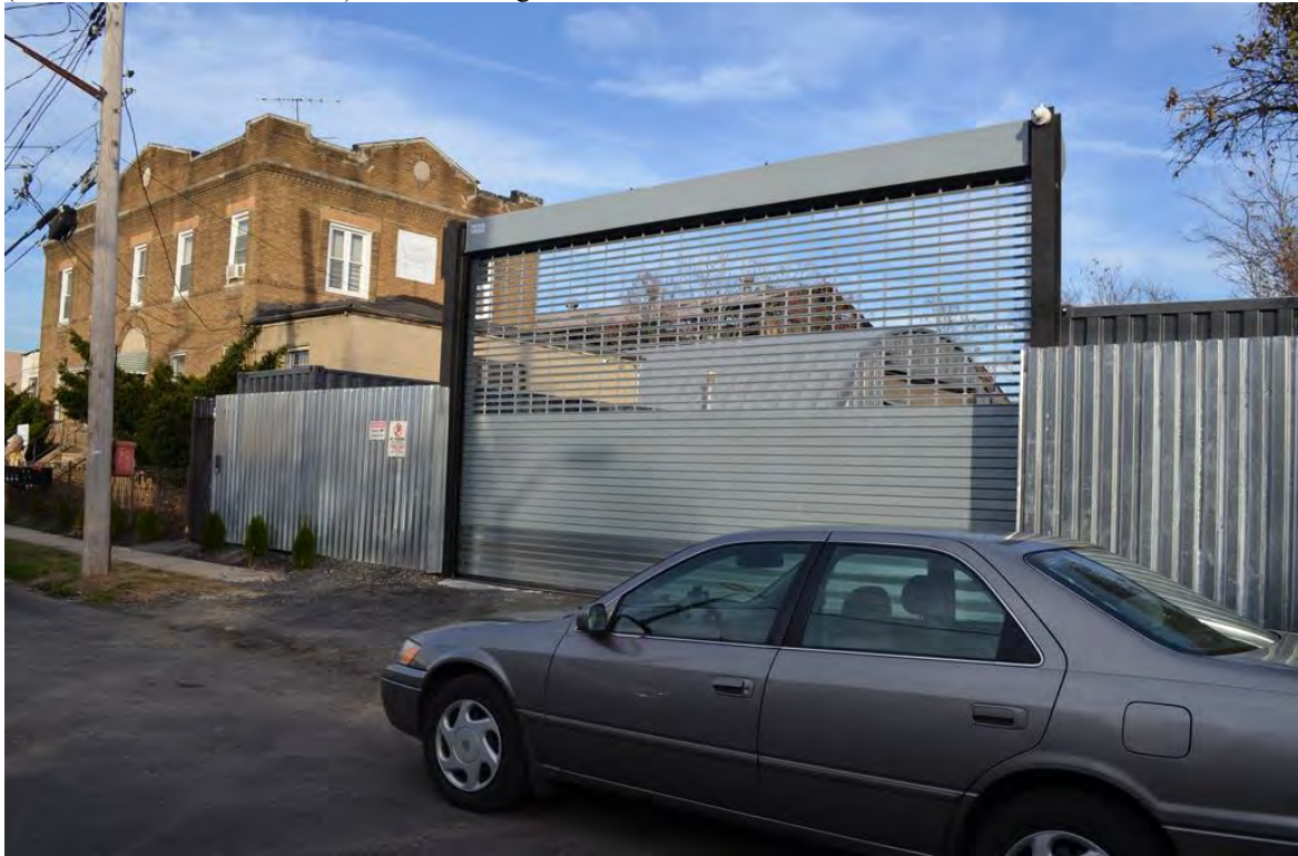
Photograph 6.13. Grandview Avenue north of and abutting the ROW. 243 Grandview Avenue on left (Block 1256, Lot 39). View looking northeast.
