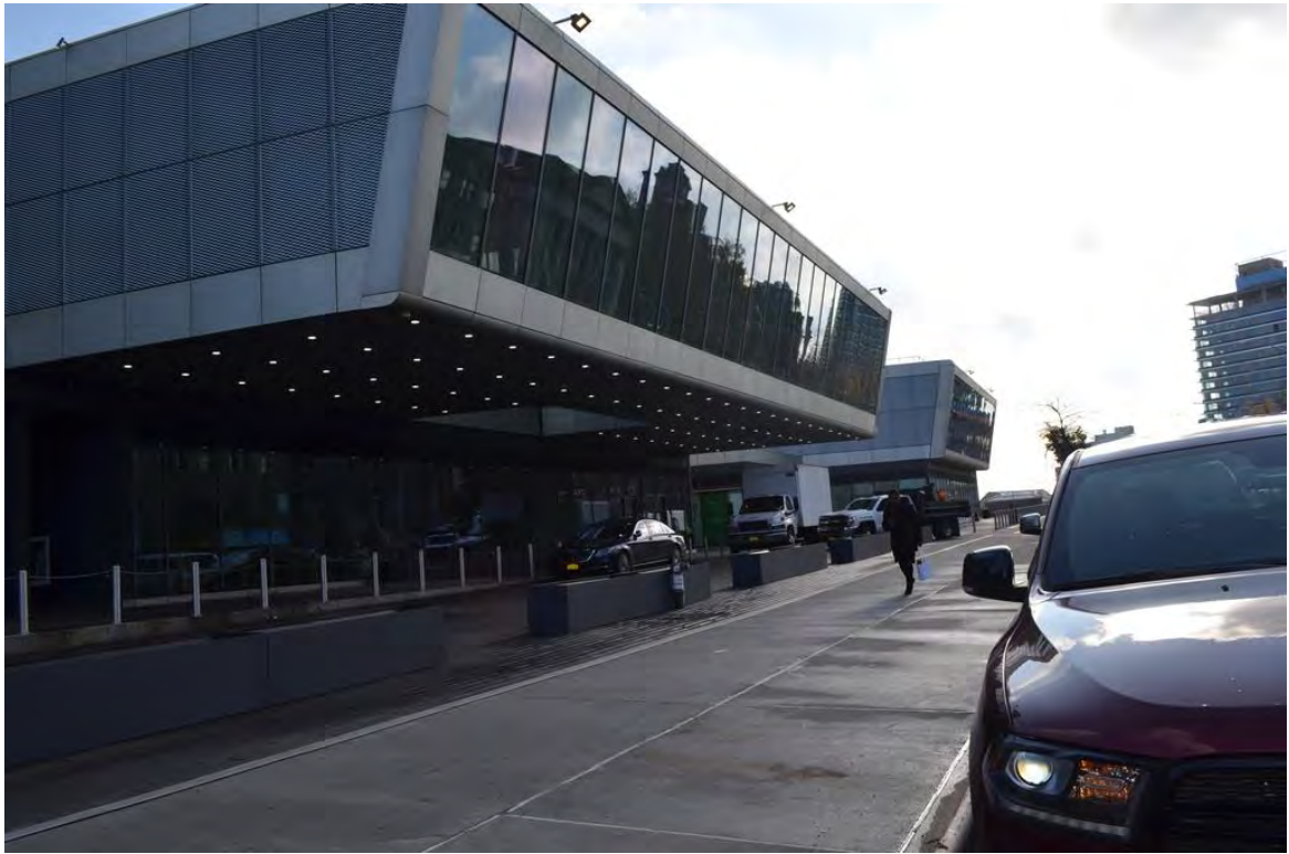
Photograph 1.2. Richmond Terrace, view looking northeast. Modern Staten Island Outlet is on left.
