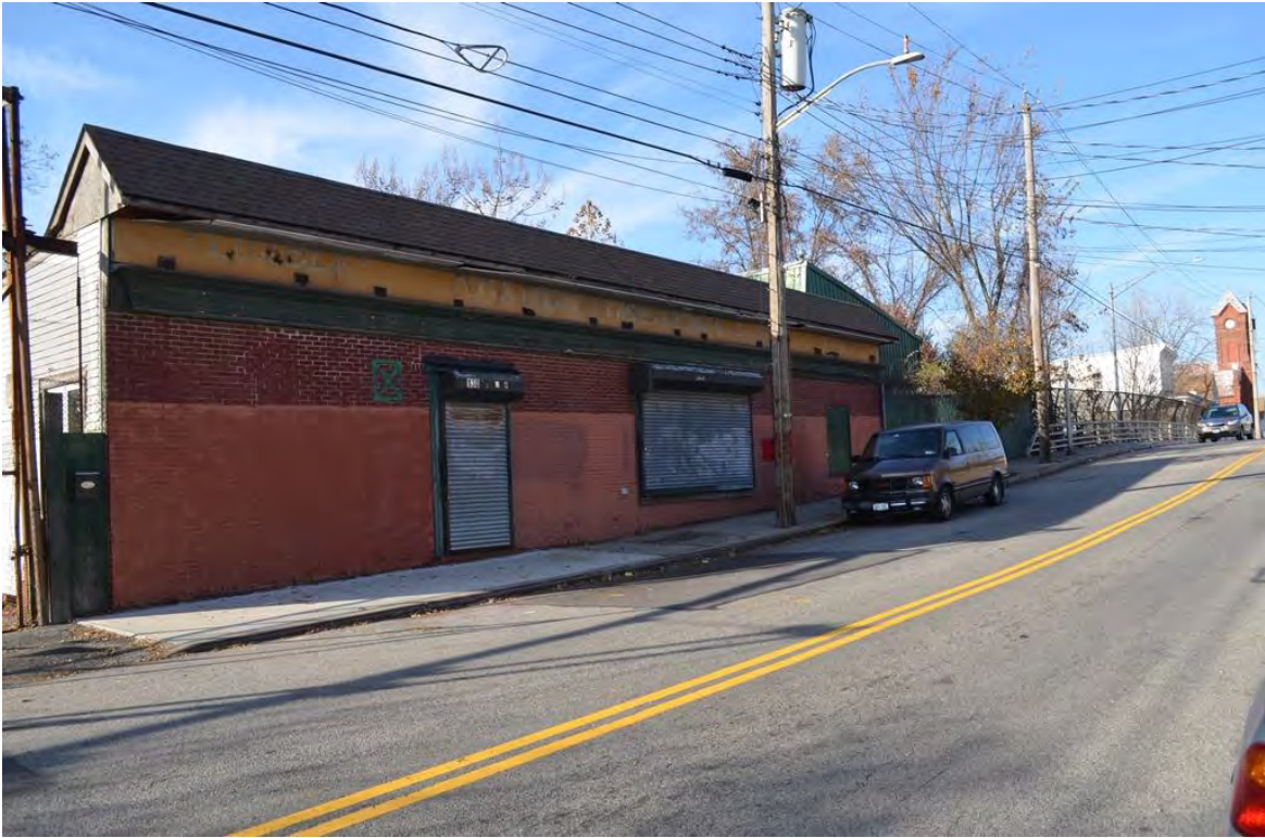
Photograph 5.50. Union Avenue south of the ROW. 130 Union Avenue (Block 1226, Lot 57). View looking northwest.
