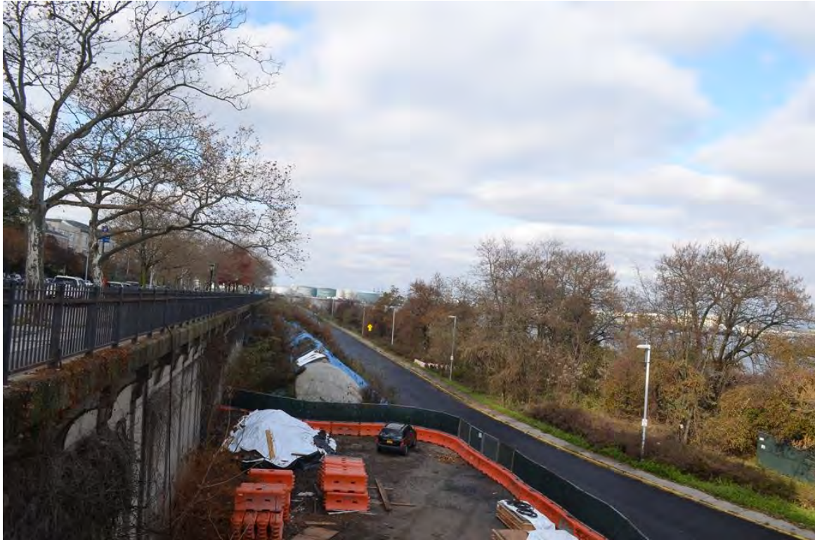
Photograph 1.5. Former railroad alignment under pavement in North Shore Waterfront Esplanade Park, with Richmond Terrace on left. View looking northwest.
