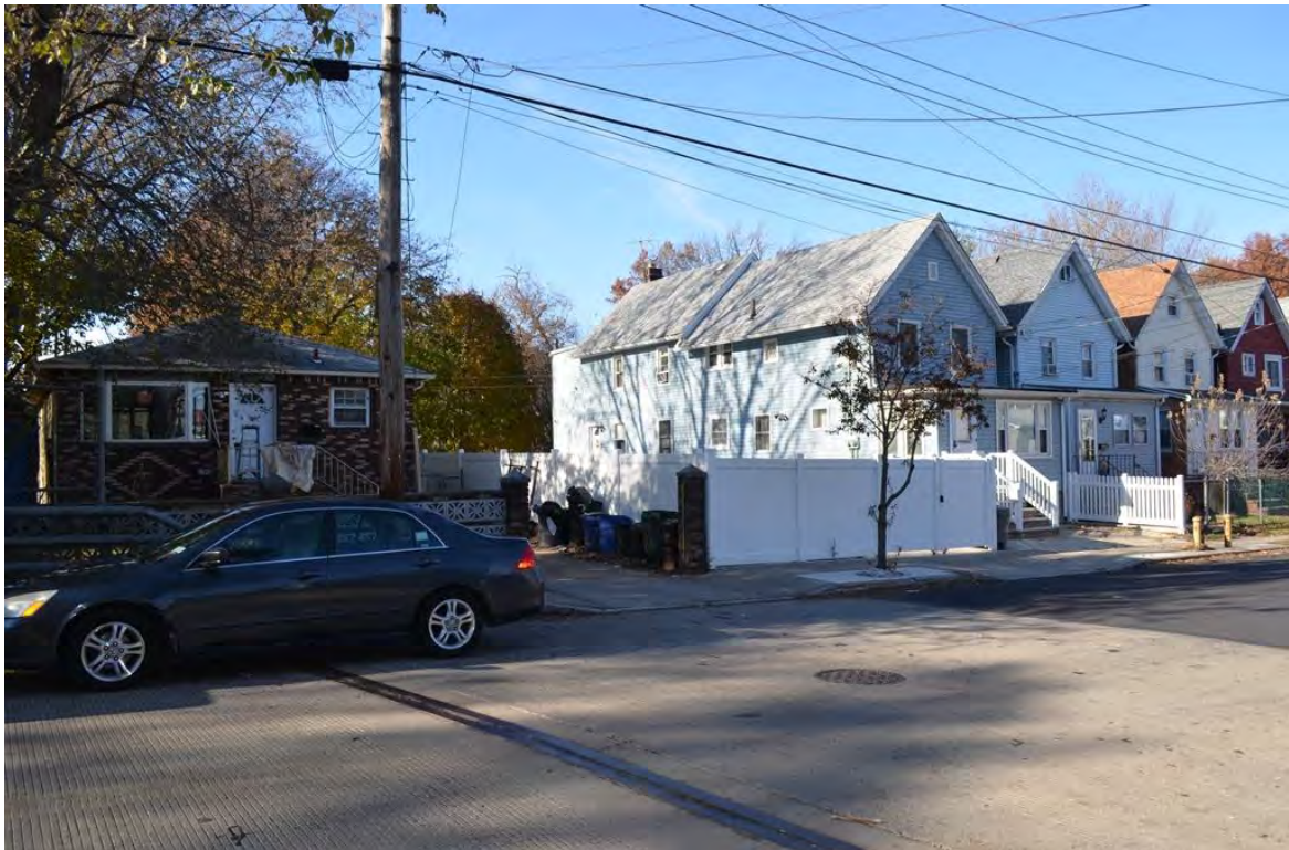
Photograph 5.26. Simonson Avenue at the northern edge of the overpass. From left: 98 and 94-88 Simonson Avenue (Block 1186, Lots 117, 115, and 114). View looking northwest.
