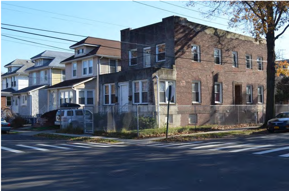
Photograph 5.33. 32 and 28 Heusden Street at the intersection of Van Name Avenue (Block 1190, Lots 28 and 30). View looking southeast.
