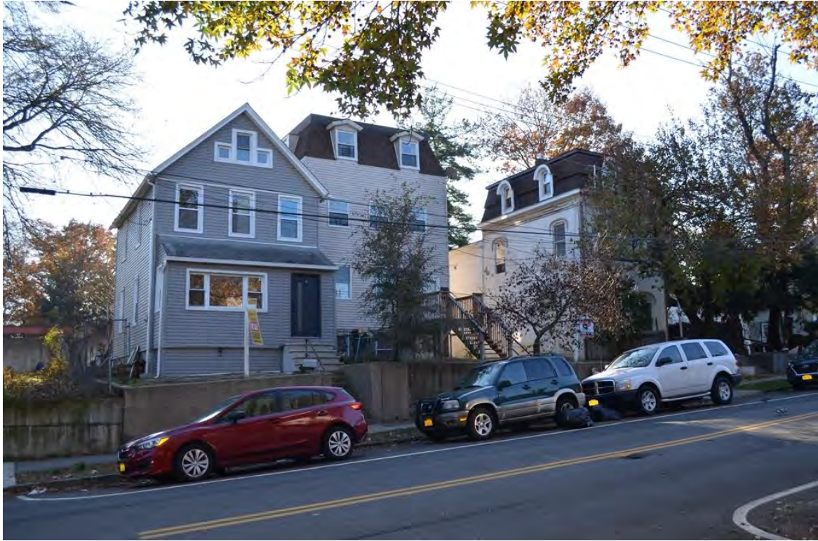
Photograph 4.9. Park Avenue south of the viaduct. 55, 57, and 61 Park Avenue (Block 1006, Lots 6, 8, and 10). View looking southeast.
