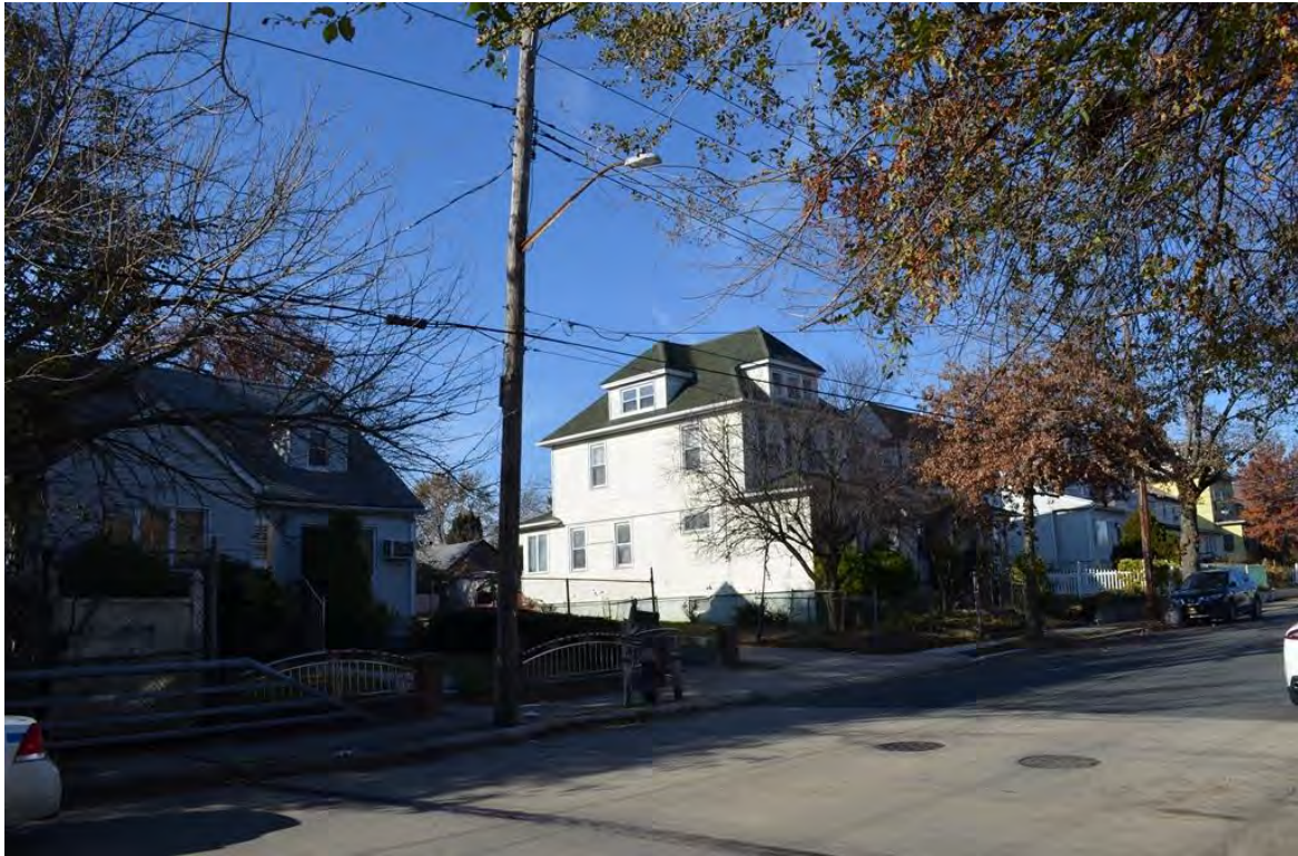
Photograph 5.38. Van Pelt Avenue north of the ROW. 92 and 88 Van Pelt Avenue (Block 1121, Lots 150 and 148). View looking northwest.
