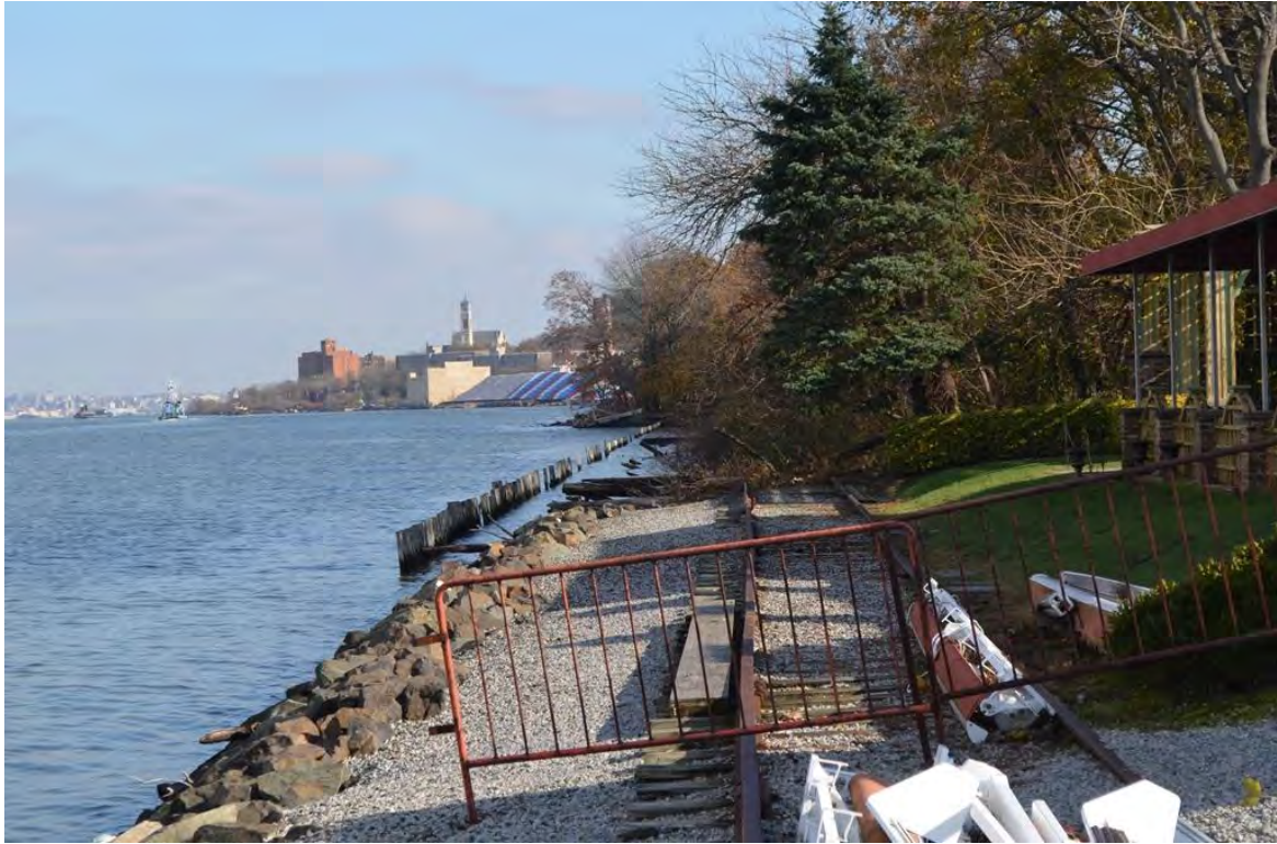
Photograph R.9. Section 2, rear of Blue Restaurant at 1115 Richmond Terrace showing the reconstructed railroad tracks. View looking east.
