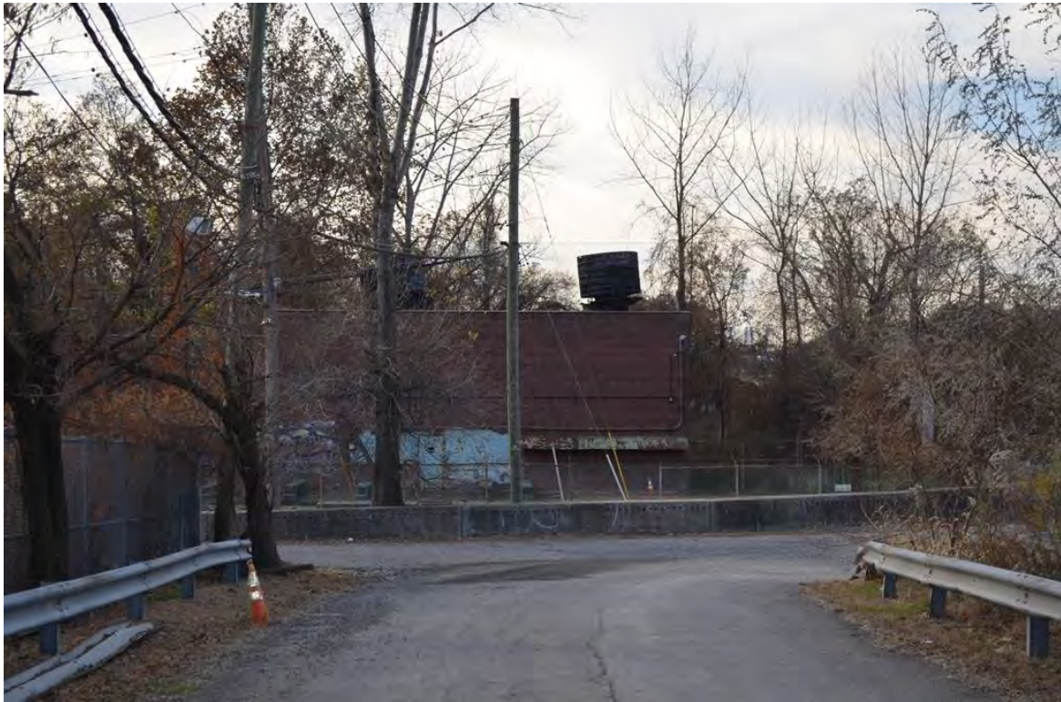
Photograph 6.10. Railroad property south of the ROW with industrial building (Block 1288, Lot 217). View looking west.
