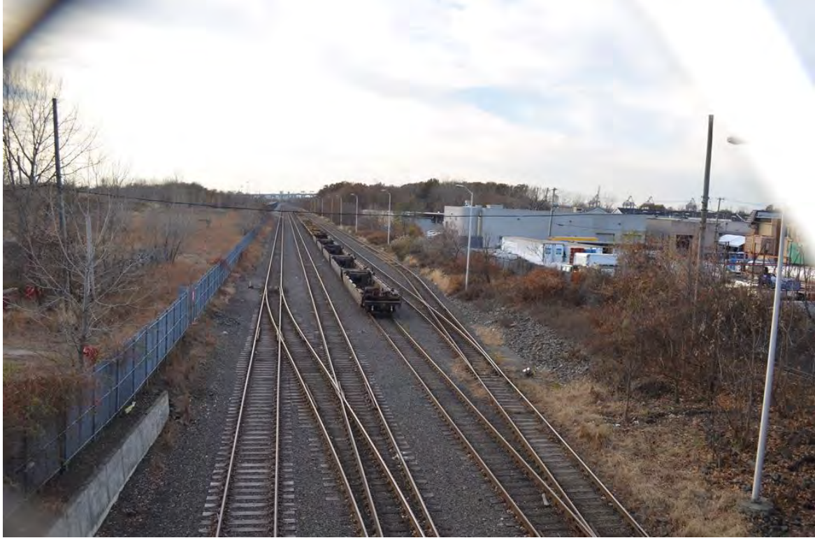
Photograph R.25. Section 6, active tracks at the South Avenue overpass. View looking west.
