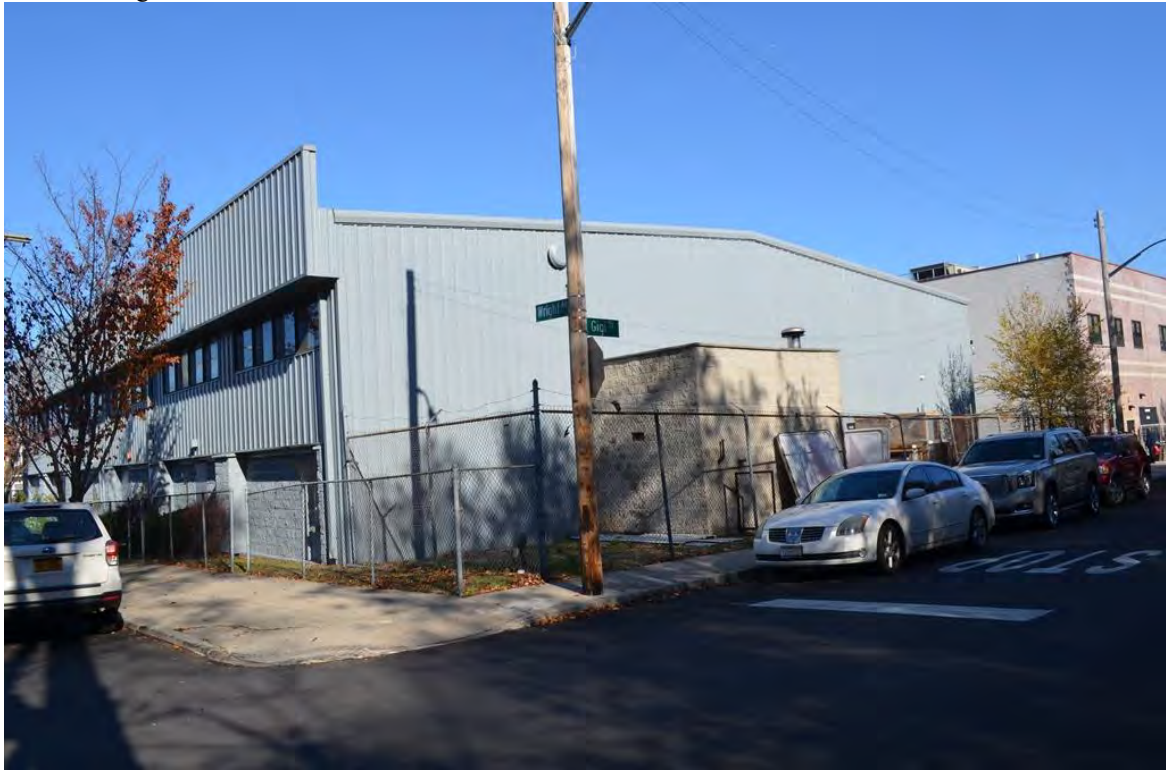
Photograph 5.18. Gigi Street and Wright Avenue north of the ROW. 93 and 91 Wright Avenue (Block 1158, Lots 1 and 7). View looking northeast.
