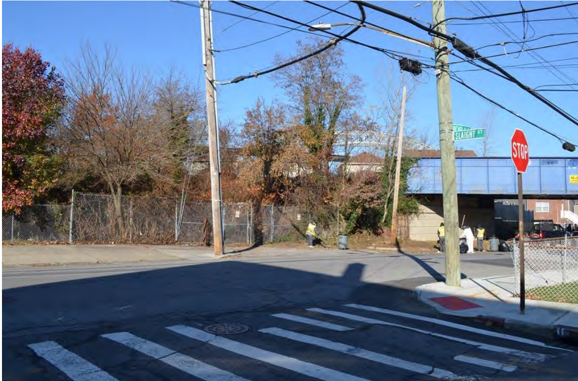
Photograph 4.41. Nicholas Avenue south of the viaduct at Slaughter Street. View looking northwest from Slaughter Street.
