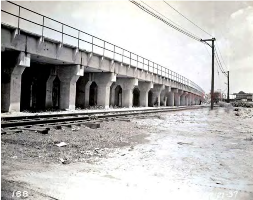
The newly constructed viaduct on the left with the older at-grade tracks on the right in 1937. Courtesy Gary Owens, http://www.gretschviking.net/GOSIRTNorthShore.htm .
