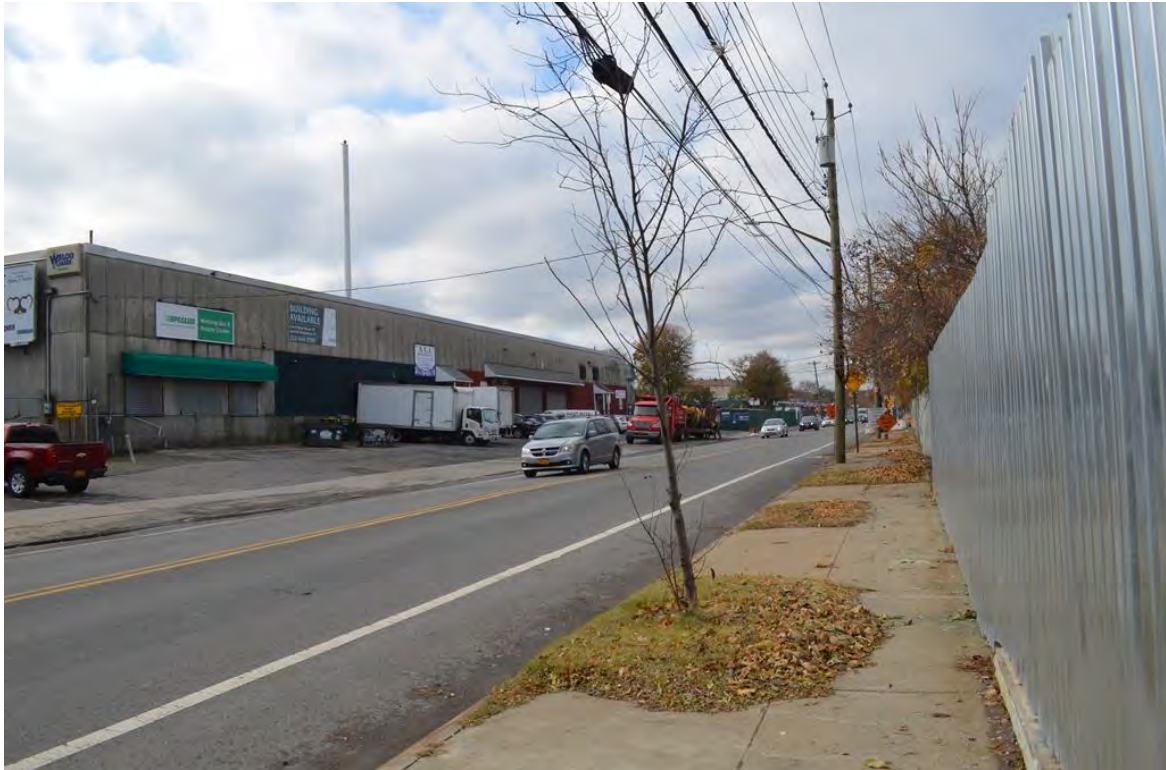
Photograph 2.6. Concrete warehouse on south side of Richmond Terrace between York Avenue and Franklin Avenue. View looking southwest.
