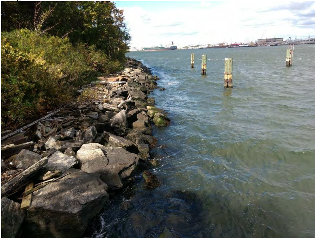
Photograph 2.26. Shoreline at Sailors' Snug Harbor. View looking west.
