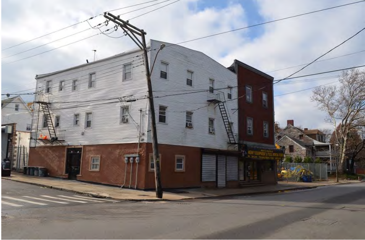
Photograph 2.11. 2 Clinton Avenue and 794 Richmond Terrace. View looking southwest.
