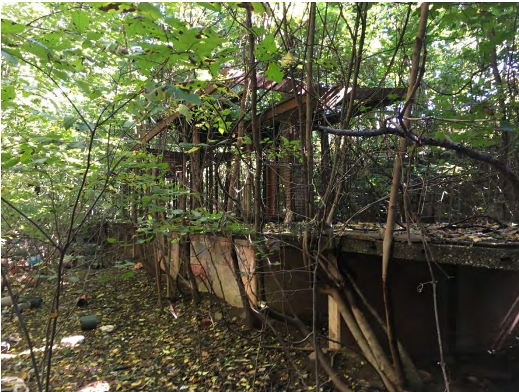
Photograph R.22. Section 5, station remnants within the open cut between De Hart Avenue and Van Pelt Avenue. View looking southeast.
