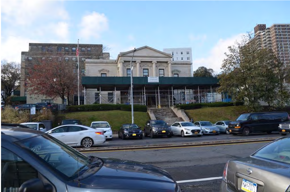
Photograph 3. Staten Island Family Courthouse, 100 Richmond Terrace. The roadway is proposed to be widened by 12 feet in front of this building, within the existing sidewalk and grassy berm. View looking northwest.
