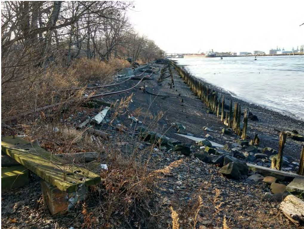
Photograph 18. Section 2, former railroad tracks along the Sailors' Snug Harbor scoured shoreline. Note the erosion of the beach. View looking west.
