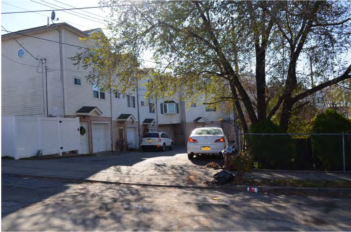
Photograph 5.7. La Salle Street at Morningstar Road north of the ROW. 15-21 Shaina Court (Block 1152, Lots, 63, 64, 66, and 67). View looking southwest.
