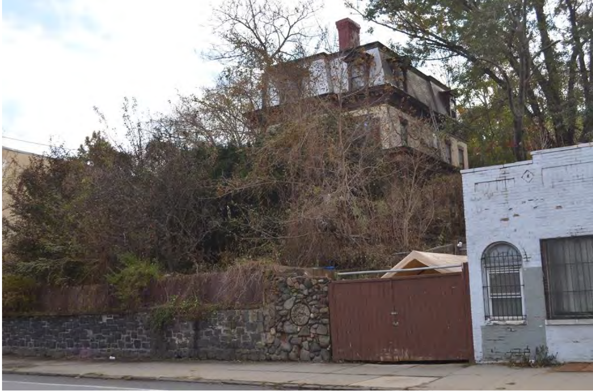
Photograph 2.5. 536 Richmond Terrace (residence on hill), view looking southeast.
