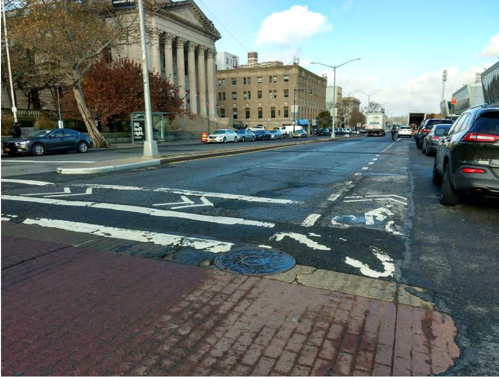
Photograph 1. Section 1, Richmond Terrace near the Staten Island Ferry Terminal. View looking northwest.
