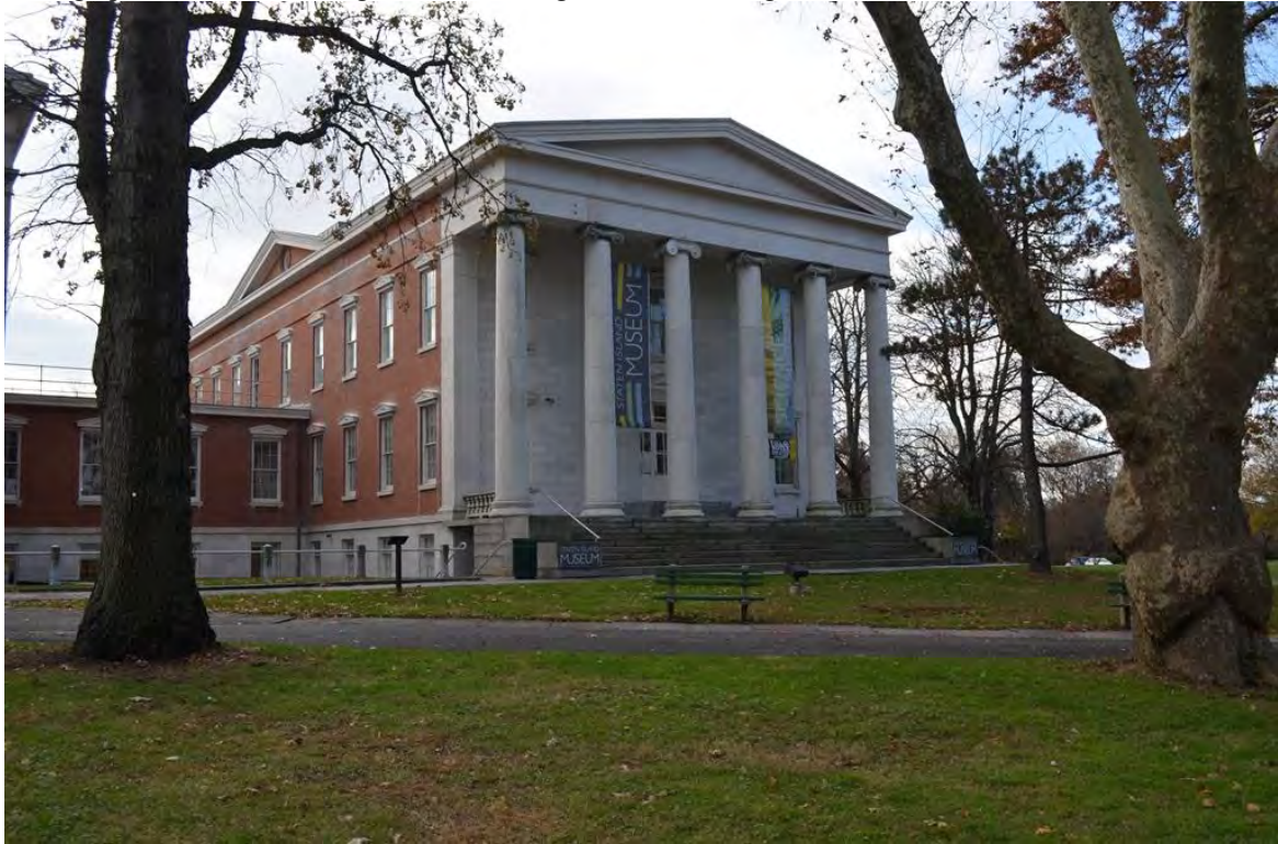
Photograph 2.20. Sailors' Snug Harbor Building A. View looking southwest.
