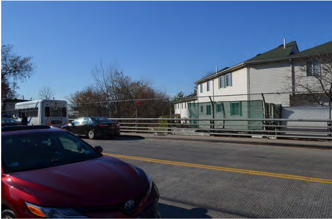
Photograph 5.6. Morningstar Road overpass above the open cut. 21 through 31 Shaina Court beyond the bridge (Block 1152, Lots 66, 68, 69, 70, 71, and 72). View looking southwest.
