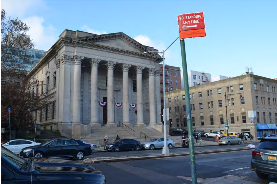
Photograph 1.7. Richmond County Courthouse, 18 Richmond Terrace. View looking northwest.
