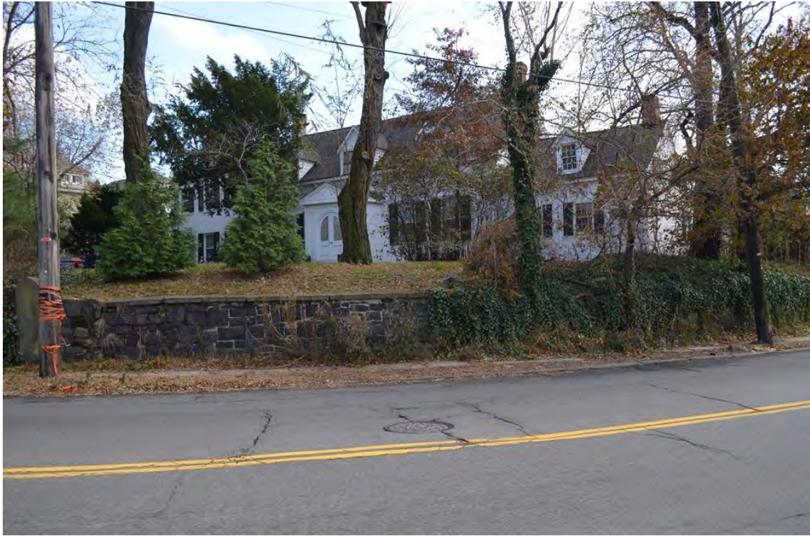
Photograph 3.10. The Kreuzer-Pelton House, 1262 Richmond Terrace, view looking southeast.
