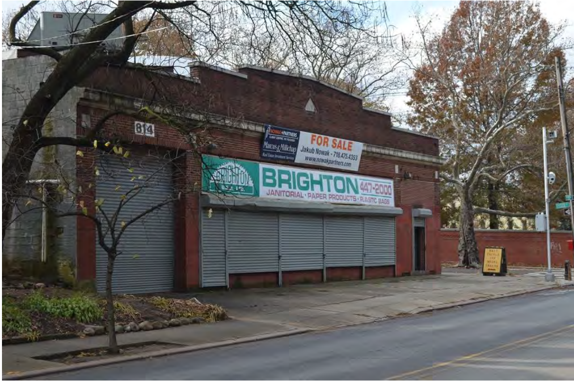
Photograph 2.13. 814 Richmond Terrace, view looking southwest.
