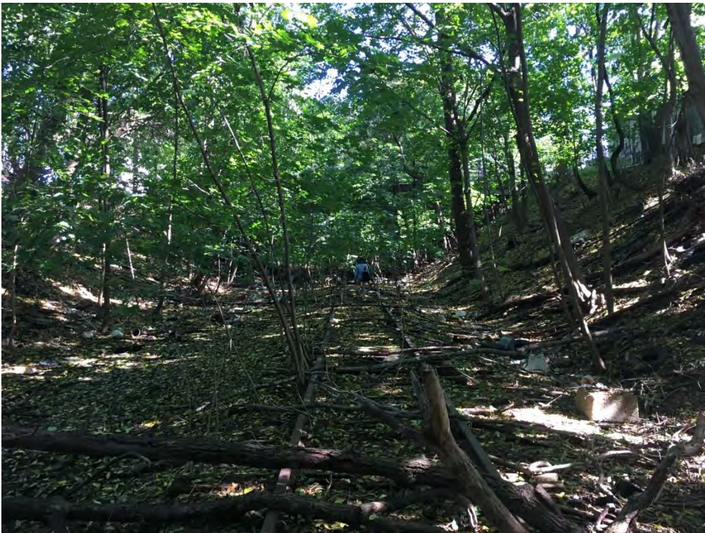
Photograph 34. Section 5, the open cut between Van Pelt Avenue and Van Name Avenue. View looking east.
