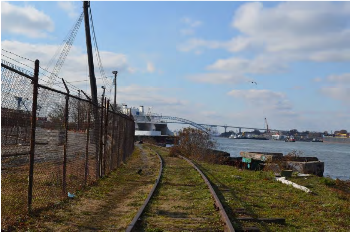
Photograph R.10. Section 2. Remains of the railroad tracks to the north of the Con Edison parking lot. View looking west.
