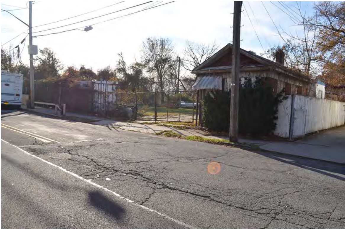
Photograph 5.46. Northern edge of the overpass at the ROW on De Hart Avenue. 100 De Hart Avenue. View looking southwest.
