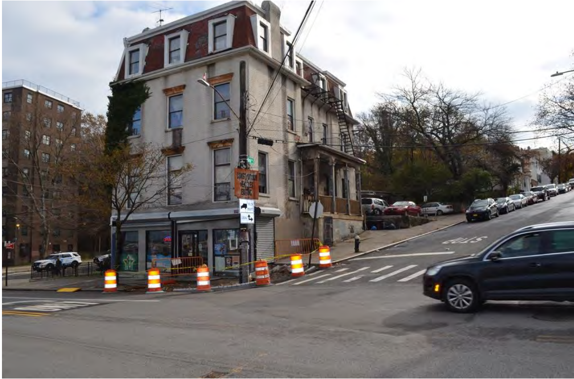
Photograph 2.3. 506 Richmond Terrace. View looking southeast.
