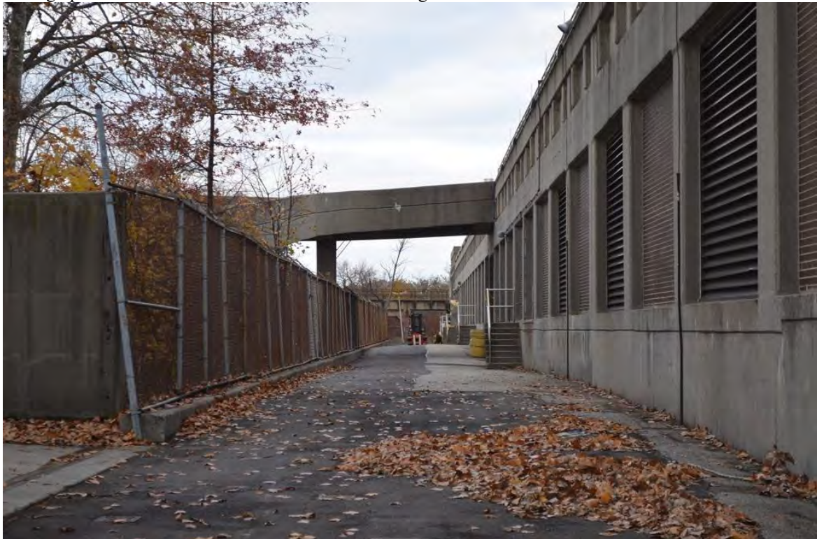
Photograph 4.4. Port Richmond Water Pollution Control Plant at 1789 Richmond Terrace with viaduct in the far background. View looking north.
