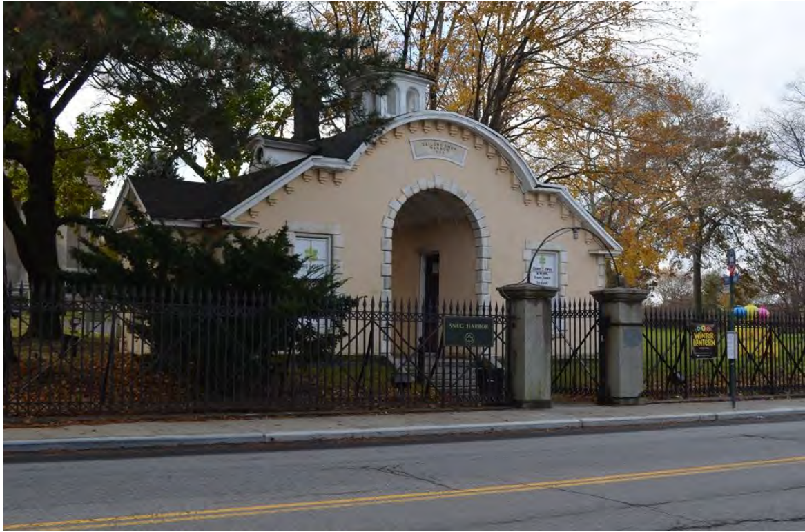
Photograph 2.15. Sailors' Snug Harbor gatehouse on Richmond Terrace. View looking southwest.
