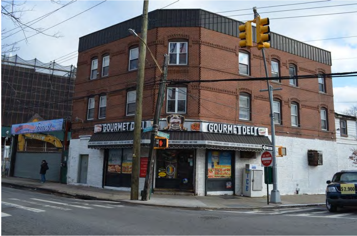
Photograph 3.13. 1410 Richmond Terrace. View looking southeast.
