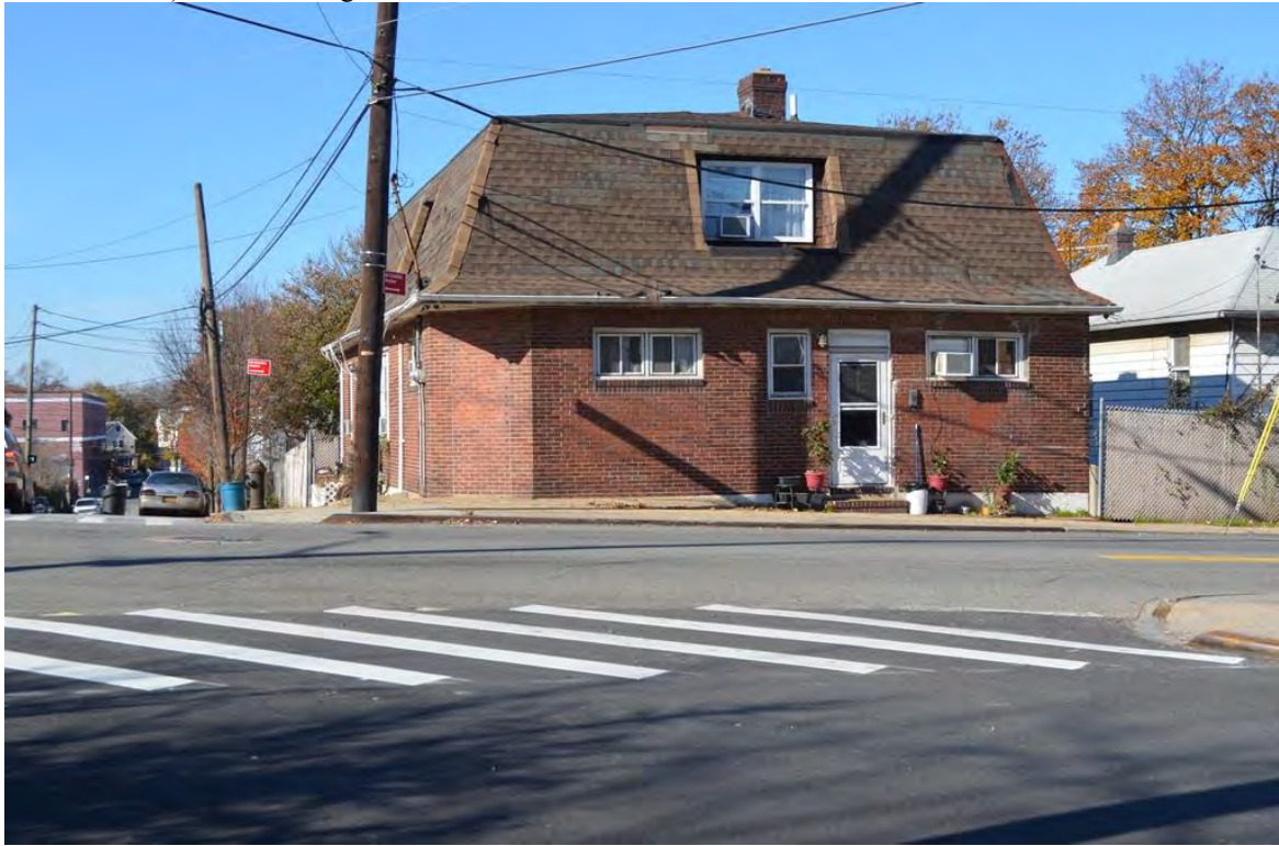
Photograph 5.8. Morningstar Road north of the ROW. 88 Morningstar Road (Block 1149, Lot 91). View looking northwest from La Salle Street.
