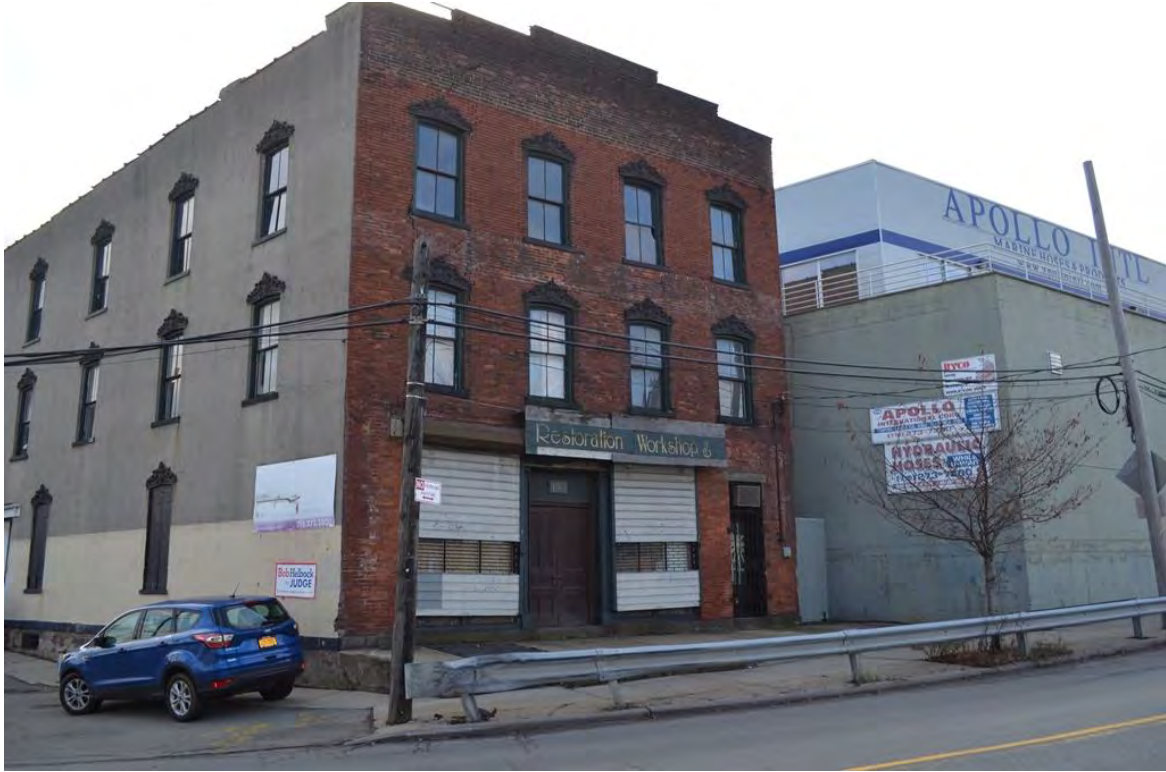
Photograph 3.14. 1550 Richmond Avenue, Restoration Workshop building. View looking southwest.
