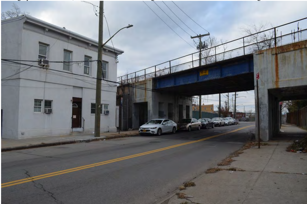
Photograph 28. Section 4, the viaduct crossing at Richmond Terrace. View looking northwest.
