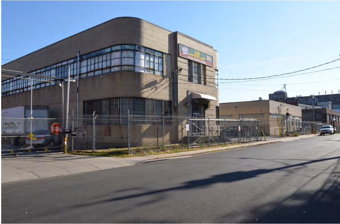
Photograph 5.23. 141 (aka 137) Lake Avenue (Block 1161, Lot 20). View looking southeast.
