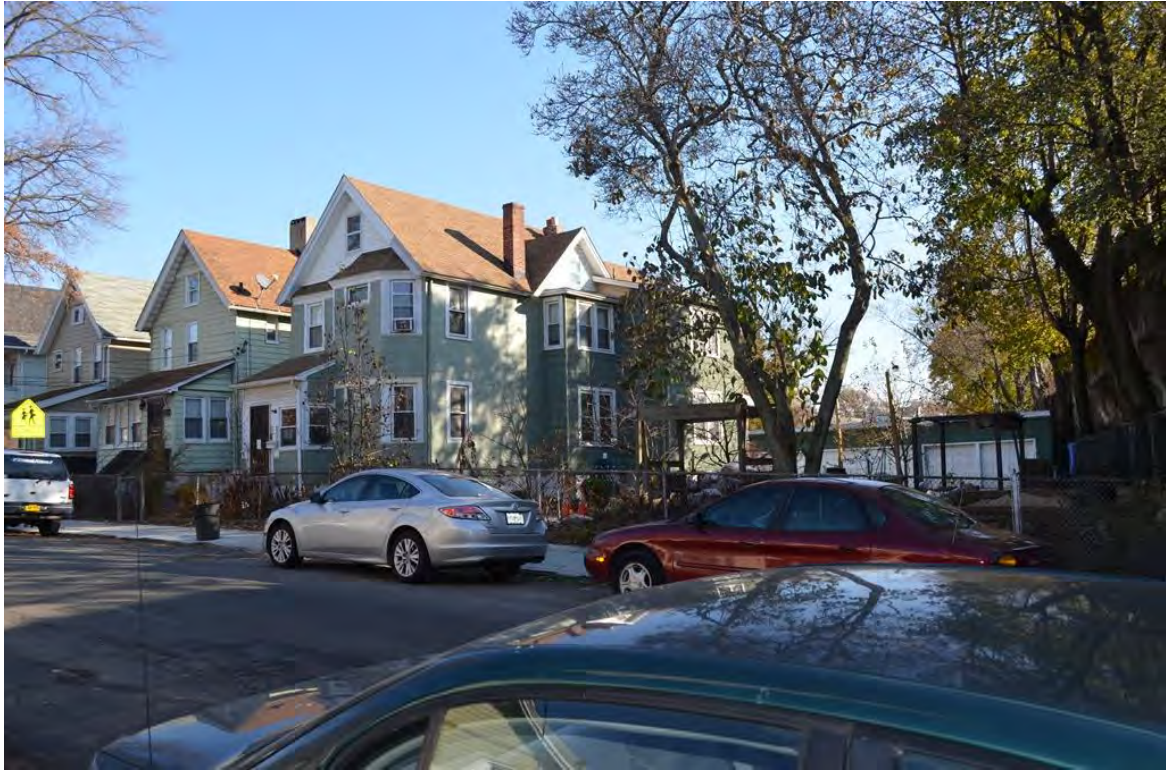
Photograph 4.29. Sharpe Avenue north of the viaduct. From right: 49, 47, and 43 Sharpe Avenue (Block 1076, Lots 28, 26, and 22). View looking northeast.
