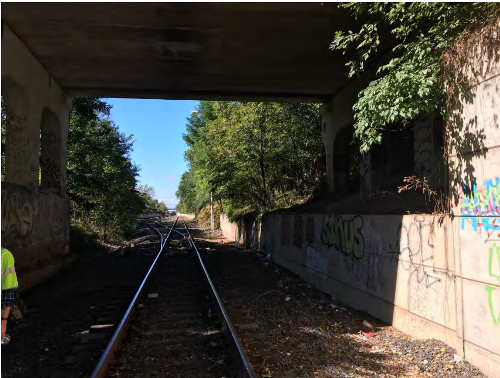
Photograph 36. Section 6, active tracks under the Harbor Road overpass. View looking west.
