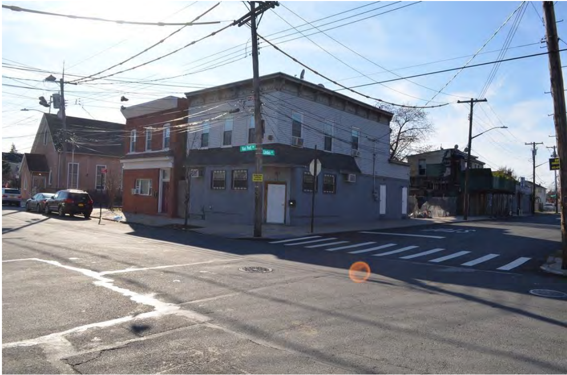
Photograph 5.36. Van Pelt and Linden Avenues. 110 and 114 Van Pelt Avenue (Block 1215, Lots 49 and 50). View looking southwest.
