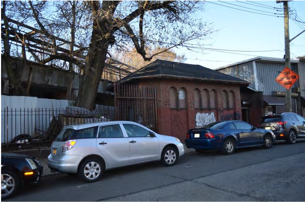
Photograph 4.10. Church Street north of the viaduct. 52-54 Church Street, circa 1931 public bathroom. View looking southwest.
