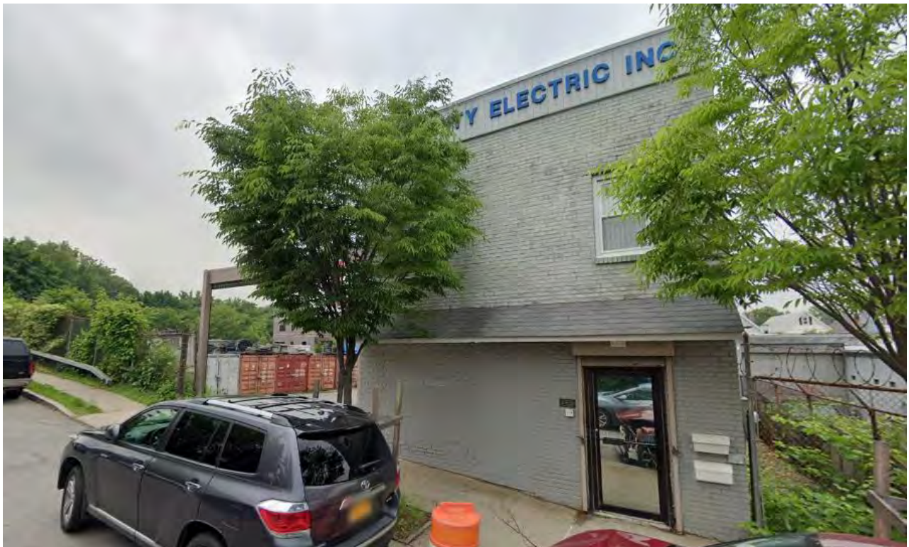
Photograph 5.16. Granite Avenue north of the ROW. 124 Granite Avenue (Block 1156, Lot 1). View looking southwest.
