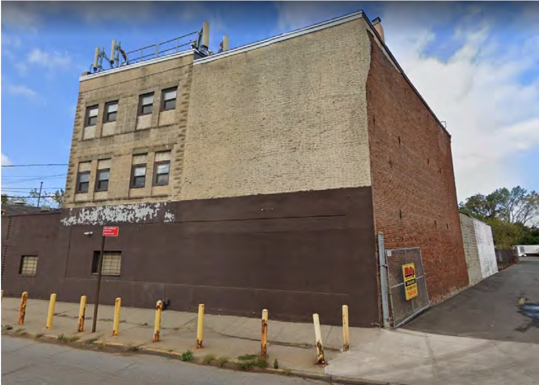
Photograph 4.2. 1689 and 1691 Richmond Terrace. View looking northwest.
