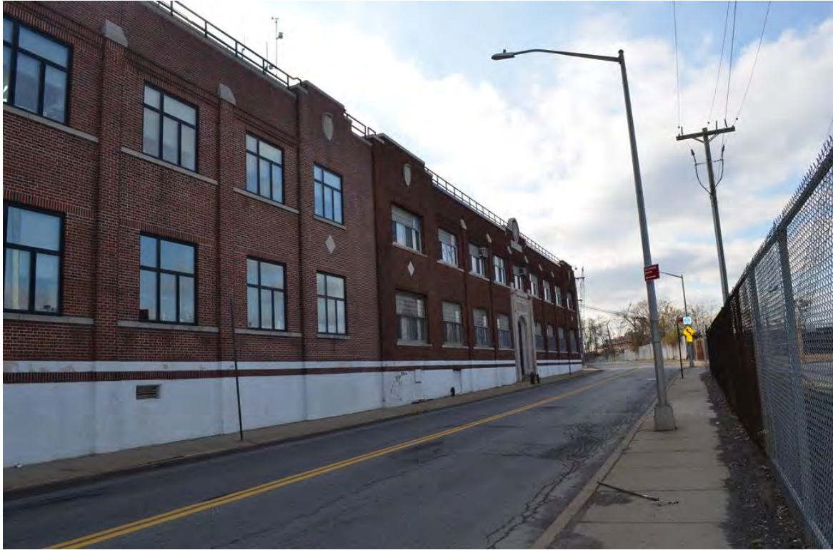
Photograph 2.33. Con Edison building on Richmond Terrace, view looking southwest near Bard Avenue.
