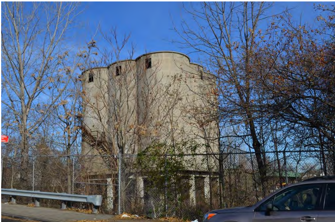
Photograph 5.54. Harbor Road south of the ROW. Coal silos at 151 Harbor Road (Block 1226, Lot 7). View looking northeast.
