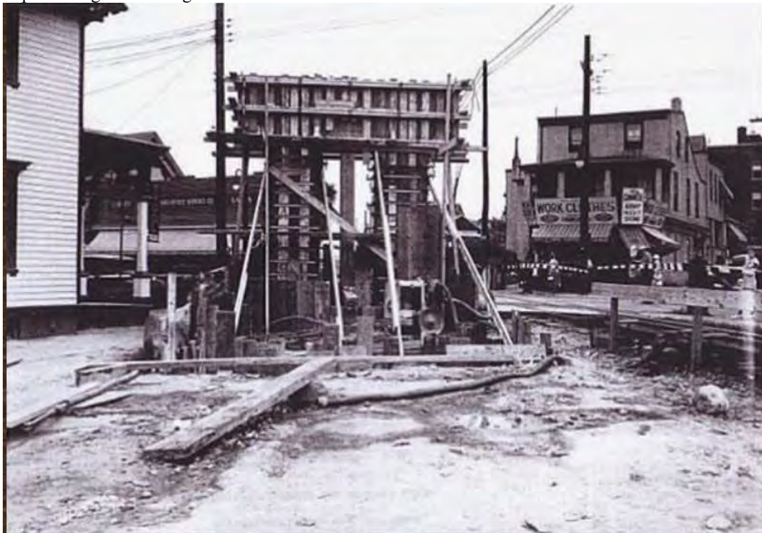
Building the viaduct at Maple Avenue in 1935. Courtesy Gary Owens, http://www.gretschviking.net/GOSIRTNorthShore.htm .
