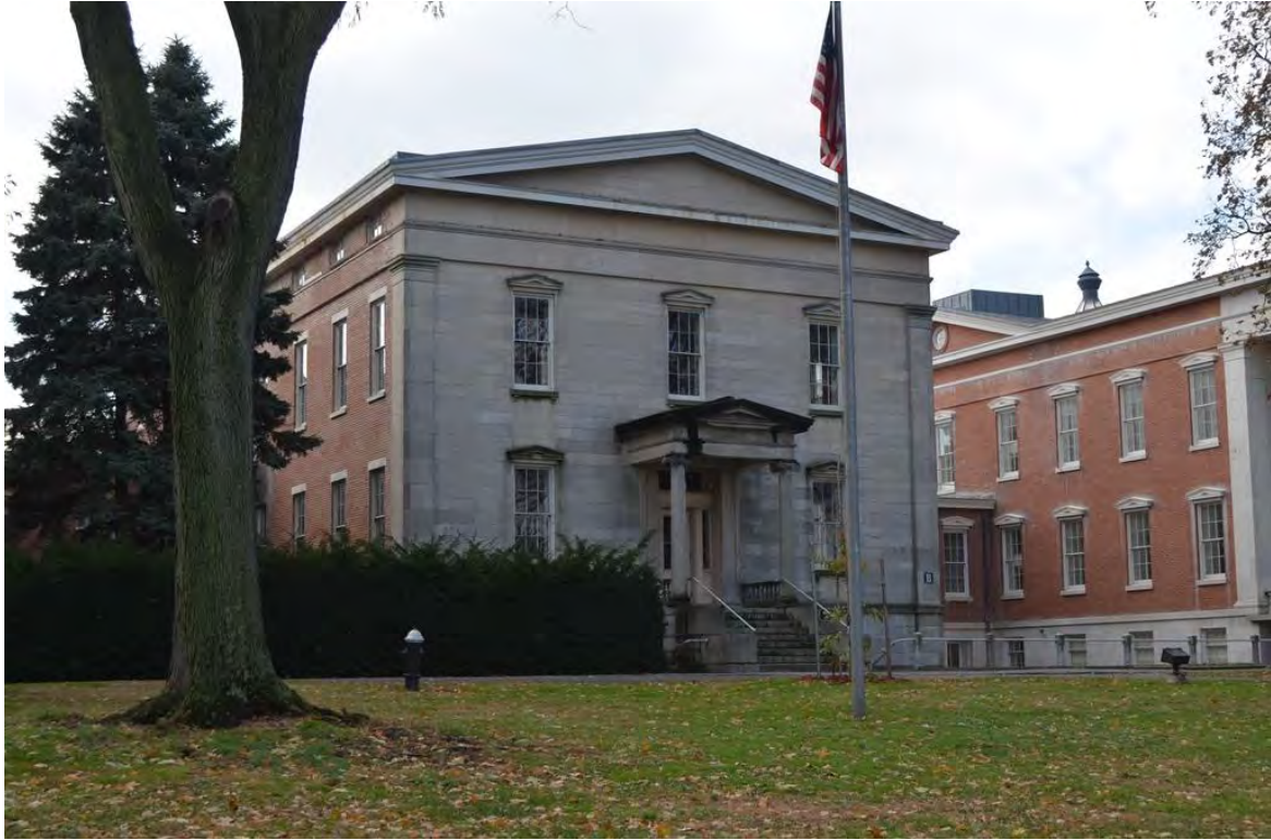
Photograph 2.19. Sailors' Snug Harbor Building B. View looking southwest.
