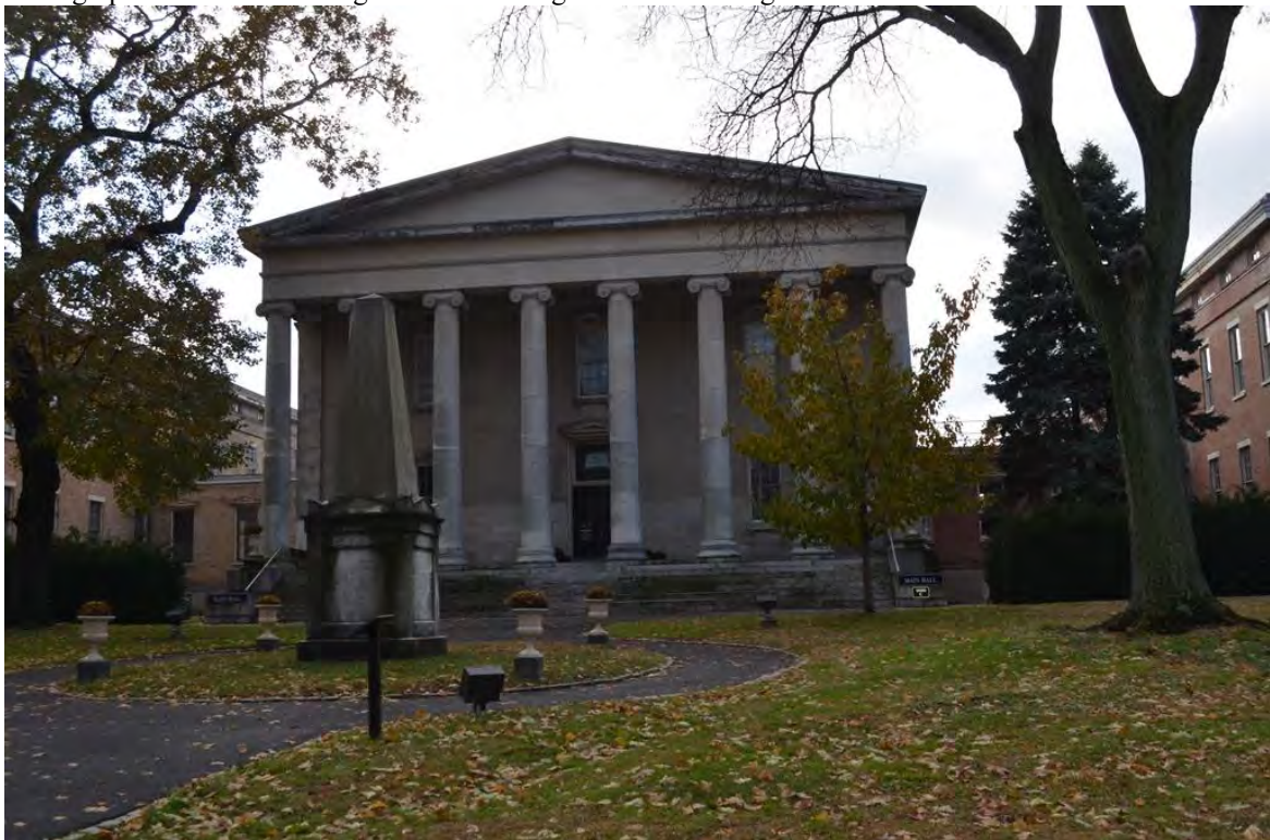
Photograph 2.18. Sailors' Snug Harbor Building C. View looking southwest.
