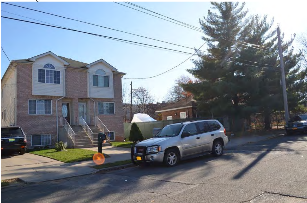
Photograph 5.12. Winant Street north of the ROW. 111 Winant Street (Block 1152, Lot 47). View looking southeast.
