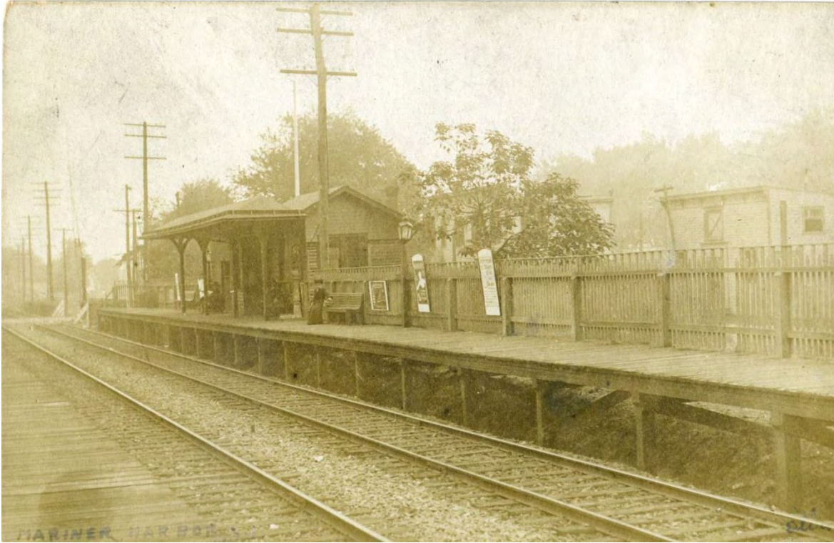
Mariners' Harbor station prior to grade elimination, undated photograph. Courtesy Staten Island Museum.
