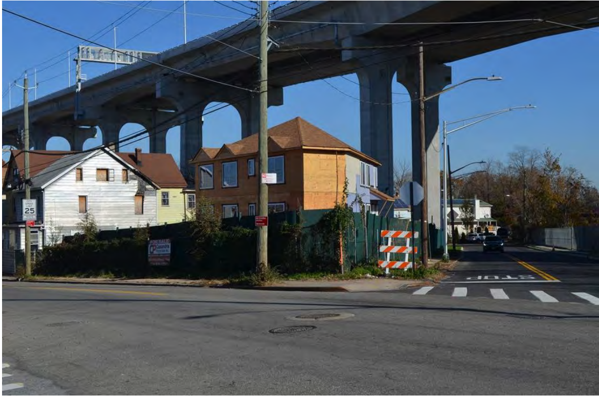
Photograph 5.9. Morningstar Road north of the ROW, with the Bayonne Bridge approach overhead. New building (no address) being constructed and 73 Morningstar Road (Block 1125, Lots 28 and 29). View looking northeast.
