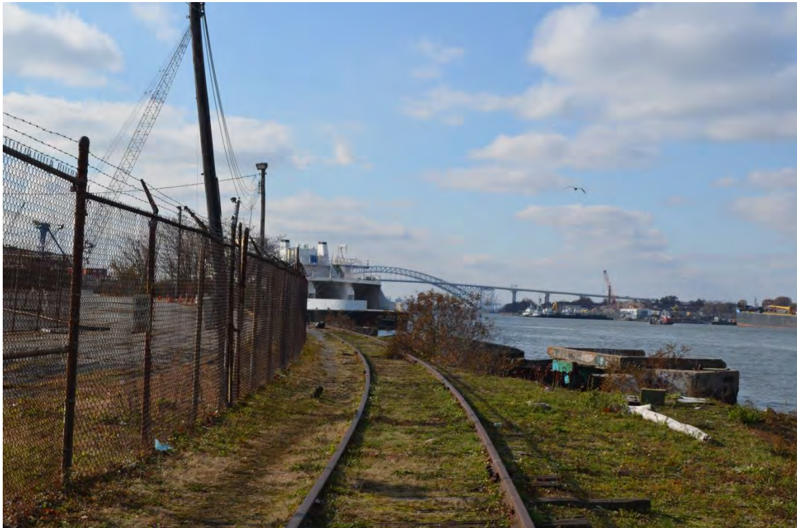
Photograph 20. Section 2, remains of the railroad tracks to the north of the Con Edison parking lot. View looking west.
