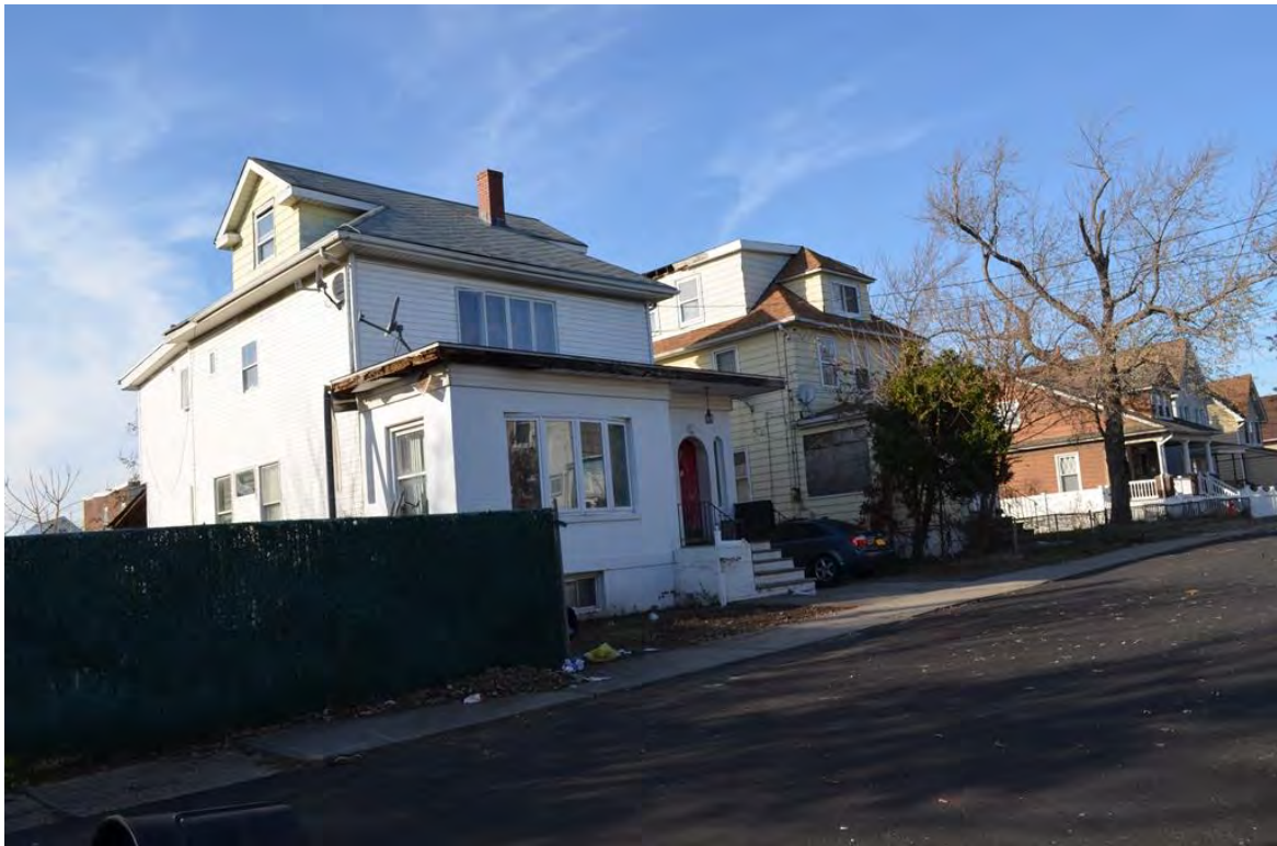
Photograph 5.40. Erastina Place north of the ROW. 98 Erastina Place (Block 1212, Lot 98). View looking northwest.
