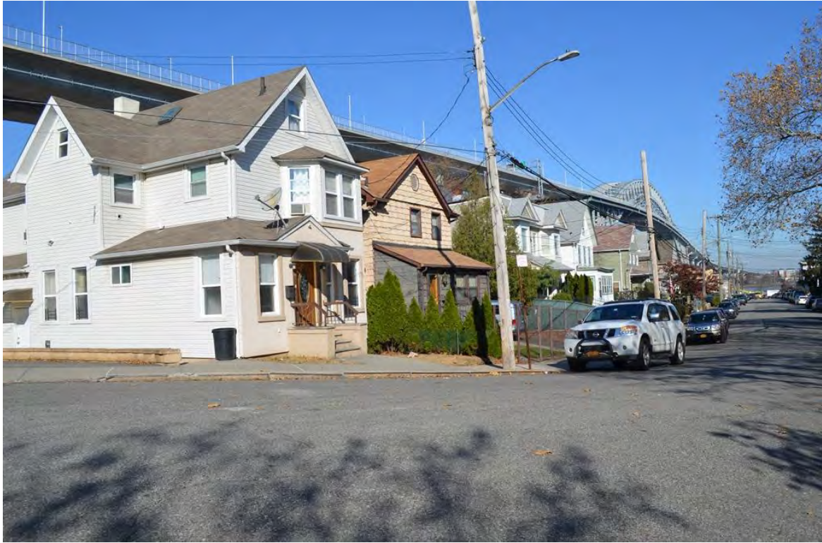
Photograph 5.1. John Street north of the ROW. From left: 94 and 92 John Street (Block 1122, Lots 108 and 105). View looking northwest.
