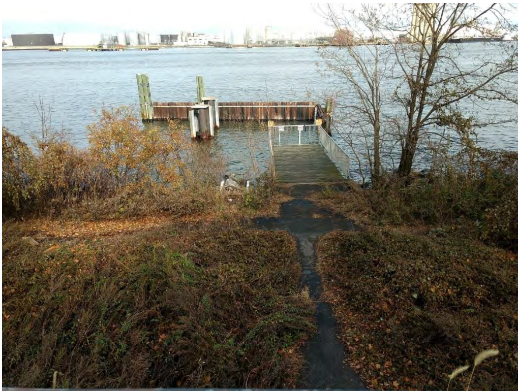
Photograph 2.24. Modern dock at Sailors' Snug Harbor on north side of Richmond Terrace. Former railroad tracks are under vegetation. View looking north.
