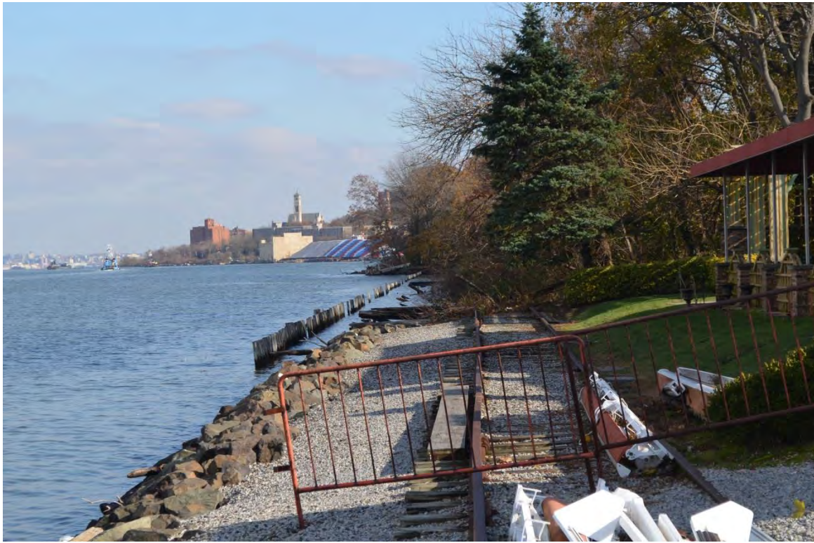
Photograph 19. Section 2, rear of Blue Restaurant at 1115 Richmond Terrace showing the reconstructed railroad tracks. View looking east.
