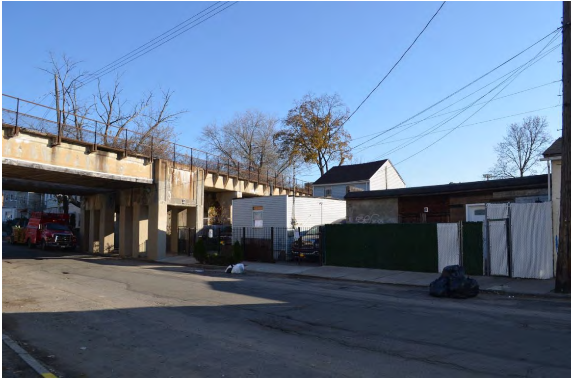
Photograph 30. Section 4, the viaduct crossing at Faber Street. View looking northeast.
