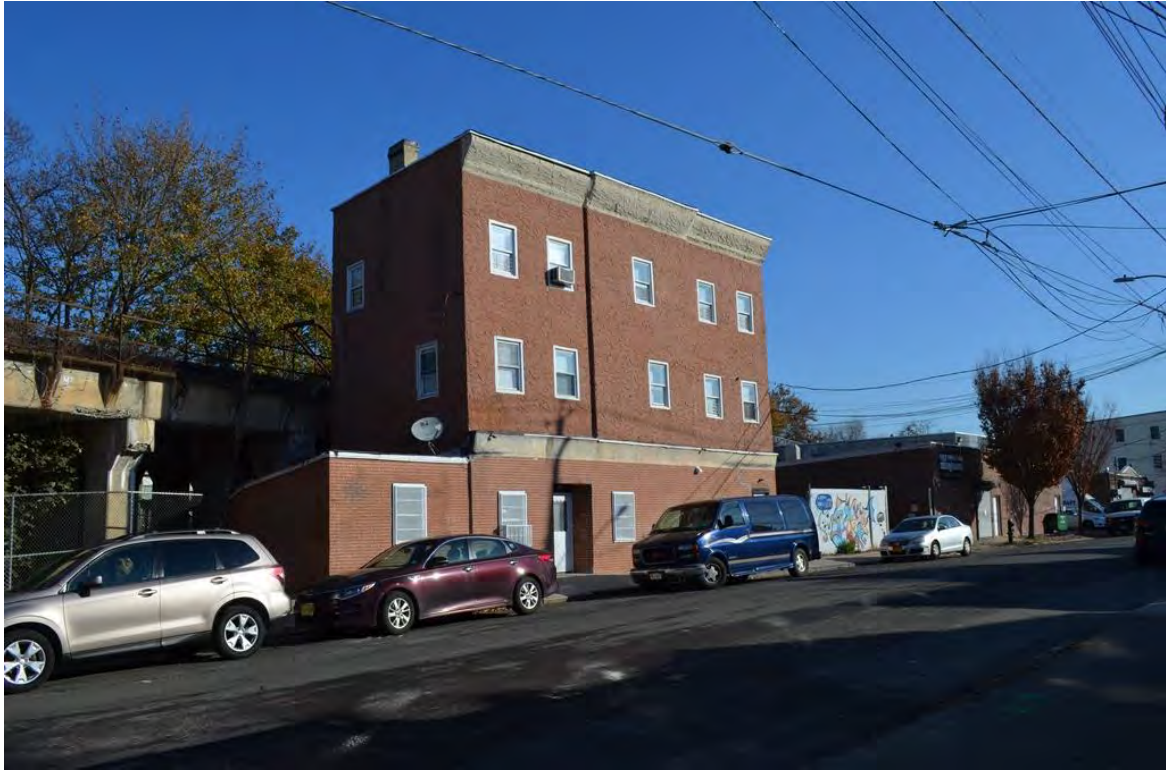
Photograph 4.33. Sharpe Avenue south of the viaduct at Grove Avenue. 97 Grove Avenue in foreground (Block 1076, Lot 14). View looking northeast.
