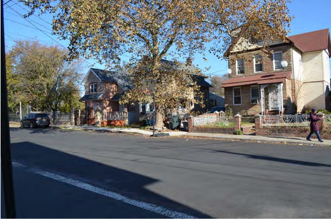
Photograph 5.27. Simonson Avenue south of the overpass. From right: 129, 125, and 121-119 Simonson Avenue (Block 1156, Lots, 32, 35, 37, and 39). View looking northeast.
