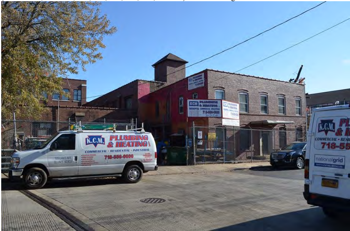
Photograph 5.22. Lake Avenue south of the overpass. 125 Lake Avenue (Block 1161, Lot 21). View looking southeast.
