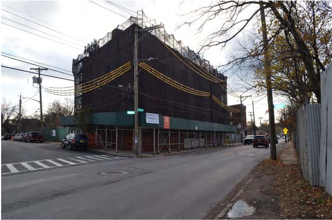
Photograph 3.12. 1390 Richmond Terrace. View looking southwest.
