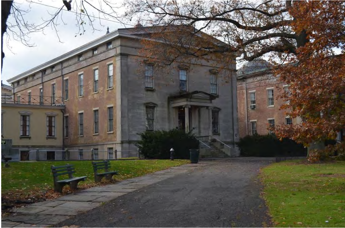
Photograph 2.17. Sailors' Snug Harbor Building D. View looking southwest.
