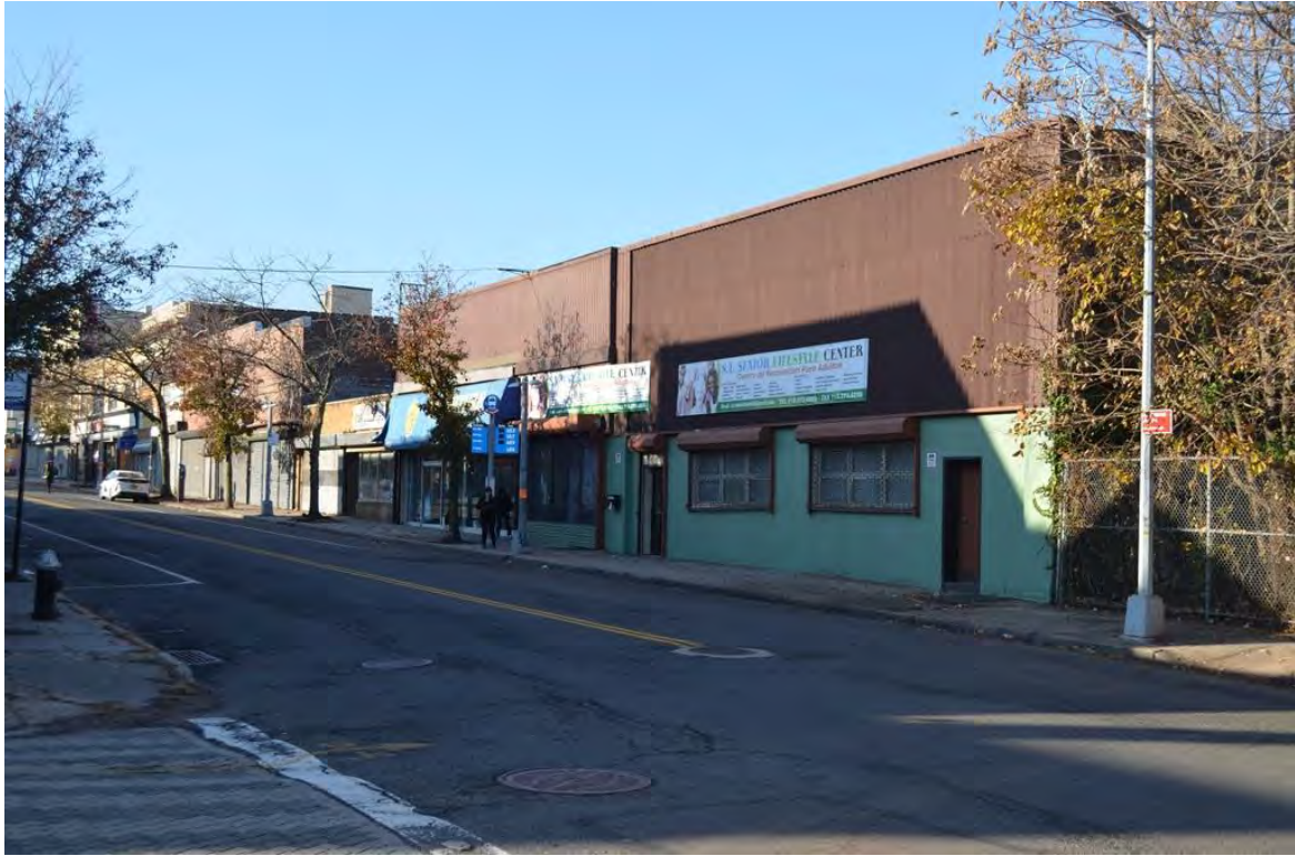
Photograph 4.15. Port Richmond Avenue, south of the viaduct. From right: 90, 98, 102, 104, 108-110, and 114 Port Richmond Avenue (Block 1073, Lots 104, 107, 110, and 116). View looking southeast.
