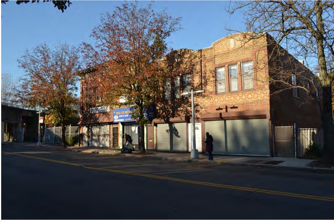
Photograph 4.13. Port Richmond Avenue north of the viaduct. From Right: 64, 68, 70, and 76 Port Richmond Avenue (Block 1073, Lots 90, 92, 93, and 94). View looking southwest.
