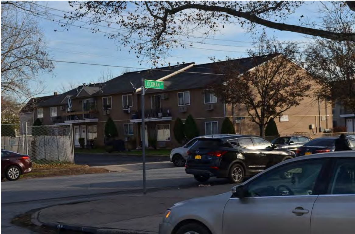
Photograph 6.5. Lockman Avenue and Lockman Loop intersection south of the ROW. 20 Lockman Loop (Block 1243, Lot 20). View looking southeast.
