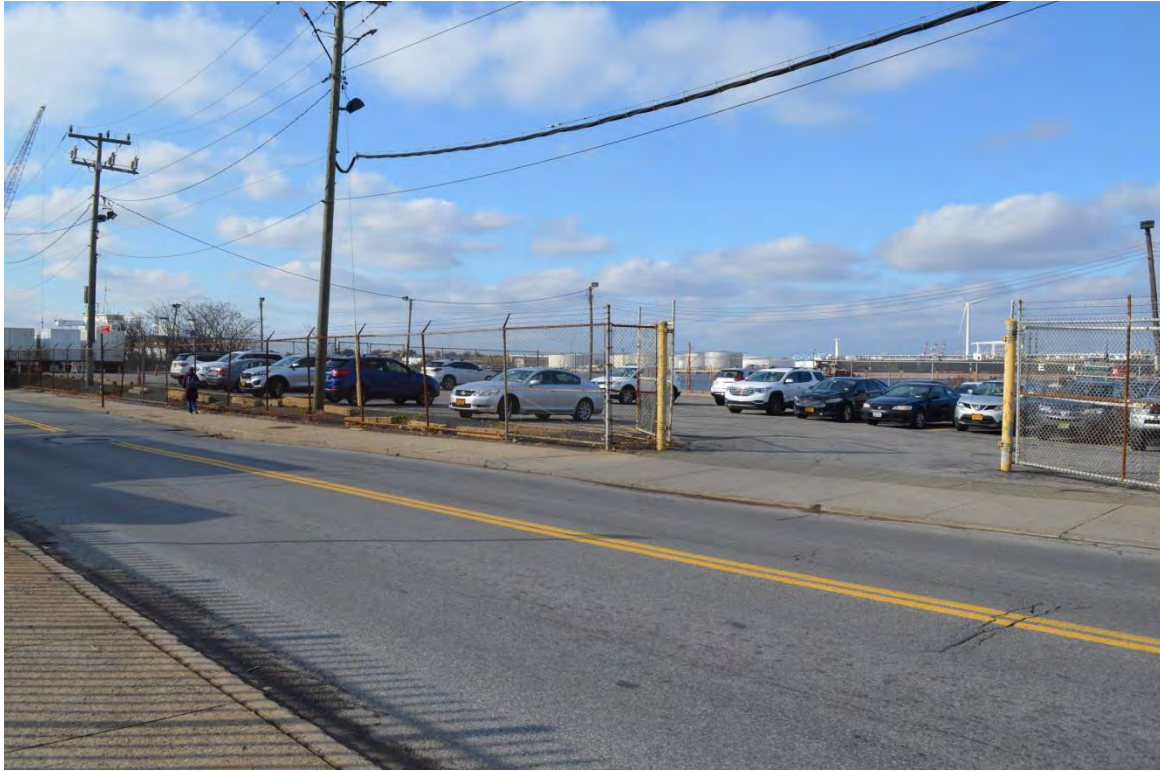
Photograph 21. Section 2, the Con Edison parking lot on the north side of Richmond Terrace that is proposed to serve first as a construction staging area and later a commuter parking lot. View looking northwest.
