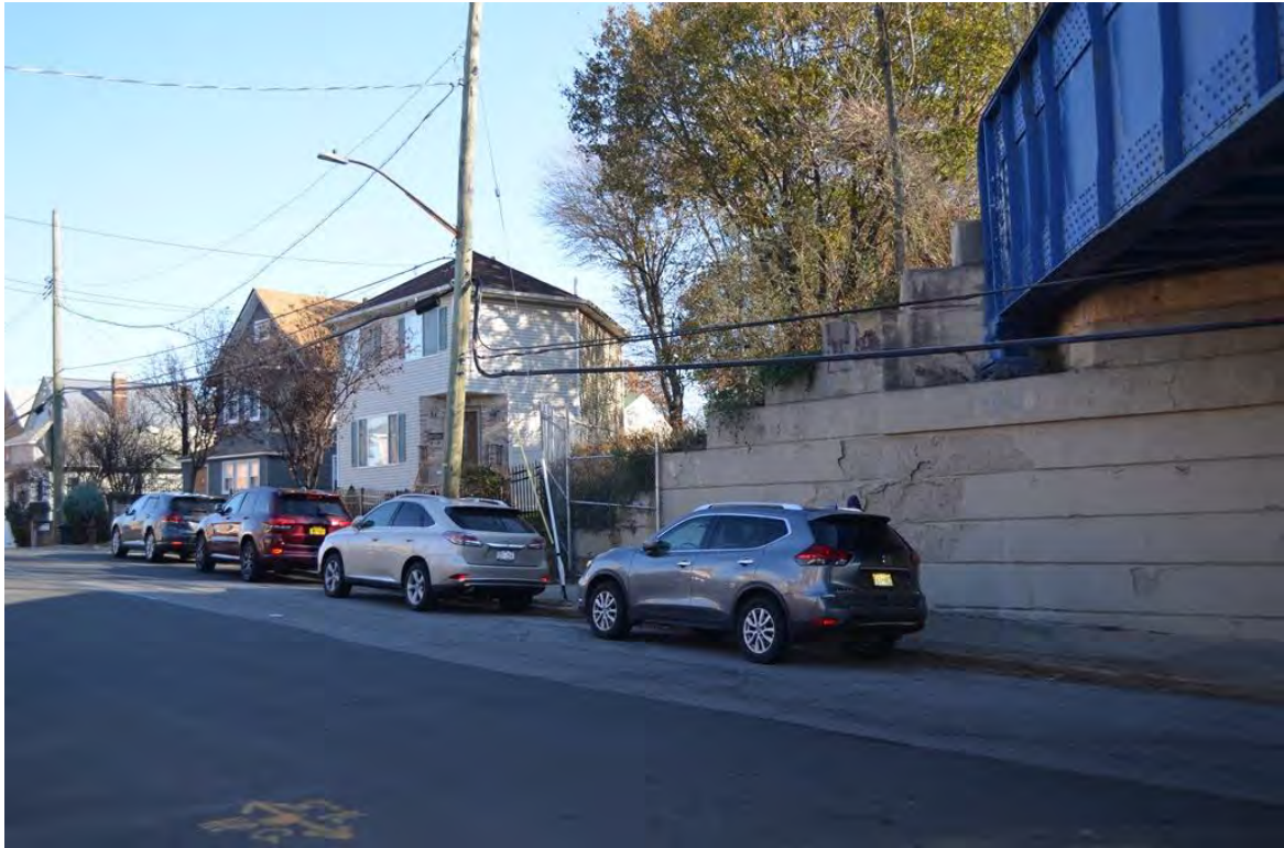
Photograph 4.42. Nicholas Avenue north of the viaduct. From right: 61, 41, and 35 Nicholas Avenue (Block 1086, Lots 32, 29, and 27). View looking northeast.
