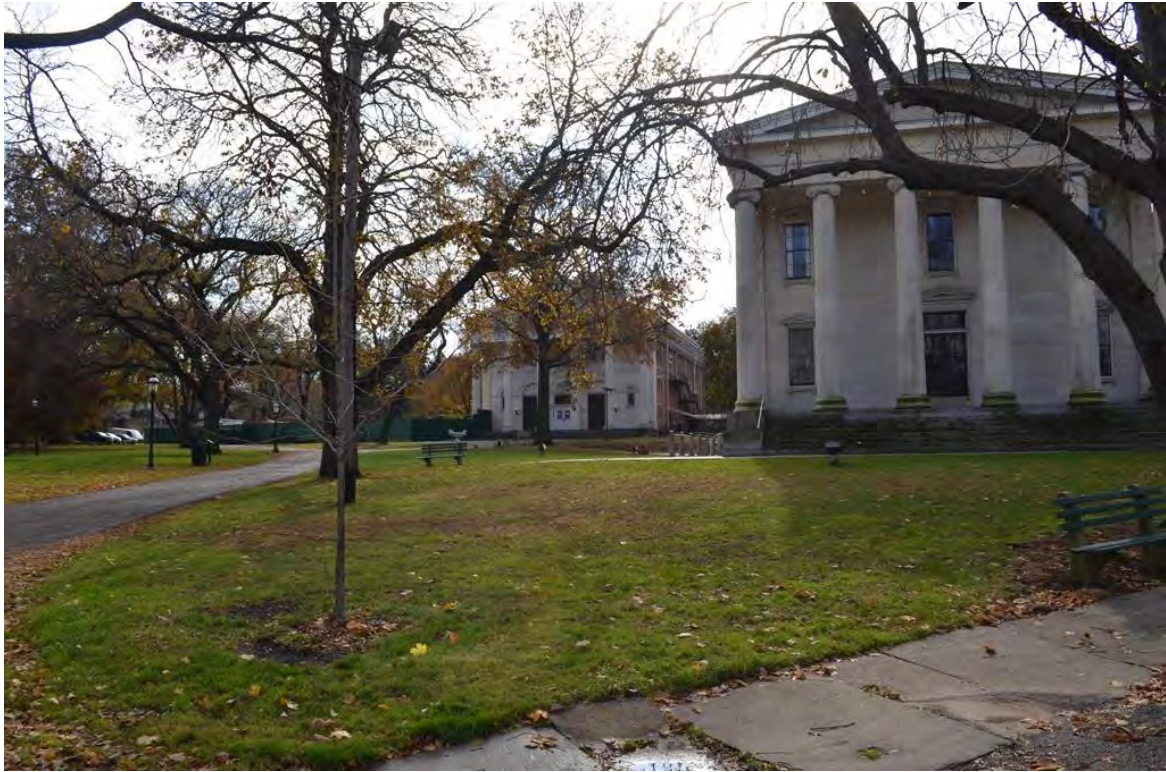
Photograph 2.16. Sailors' Snug Harbor Buildings T (left background) and E (right). View looking southwest.
