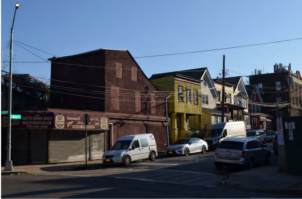
Photograph 4.17. Port Richmond Avenue at Ann Street, south of the viaduct. From left: 81 Port Richmond Avenue and 103, 99, 97, 95, 91, and 85 Ann Street (Block 1004, Lots 40, 37, 37, 36, 35, and 32). View looking northeast.
