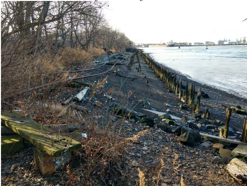
Photograph R.8. Section 2, former railroad tracks along the Sailors' Snug Harbor scoured shoreline. Note the erosion of the beach. View looking west.
