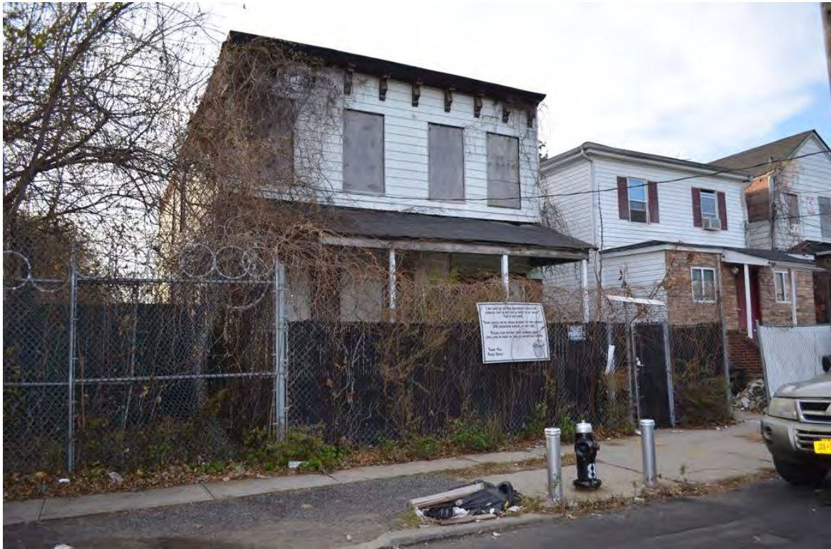
Photograph 6.12. Grandview Avenue north of and abutting the ROW. From left: 246 and 244 Grandview Avenue (Block 1257, Lots 83 and 72). View looking northwest.
