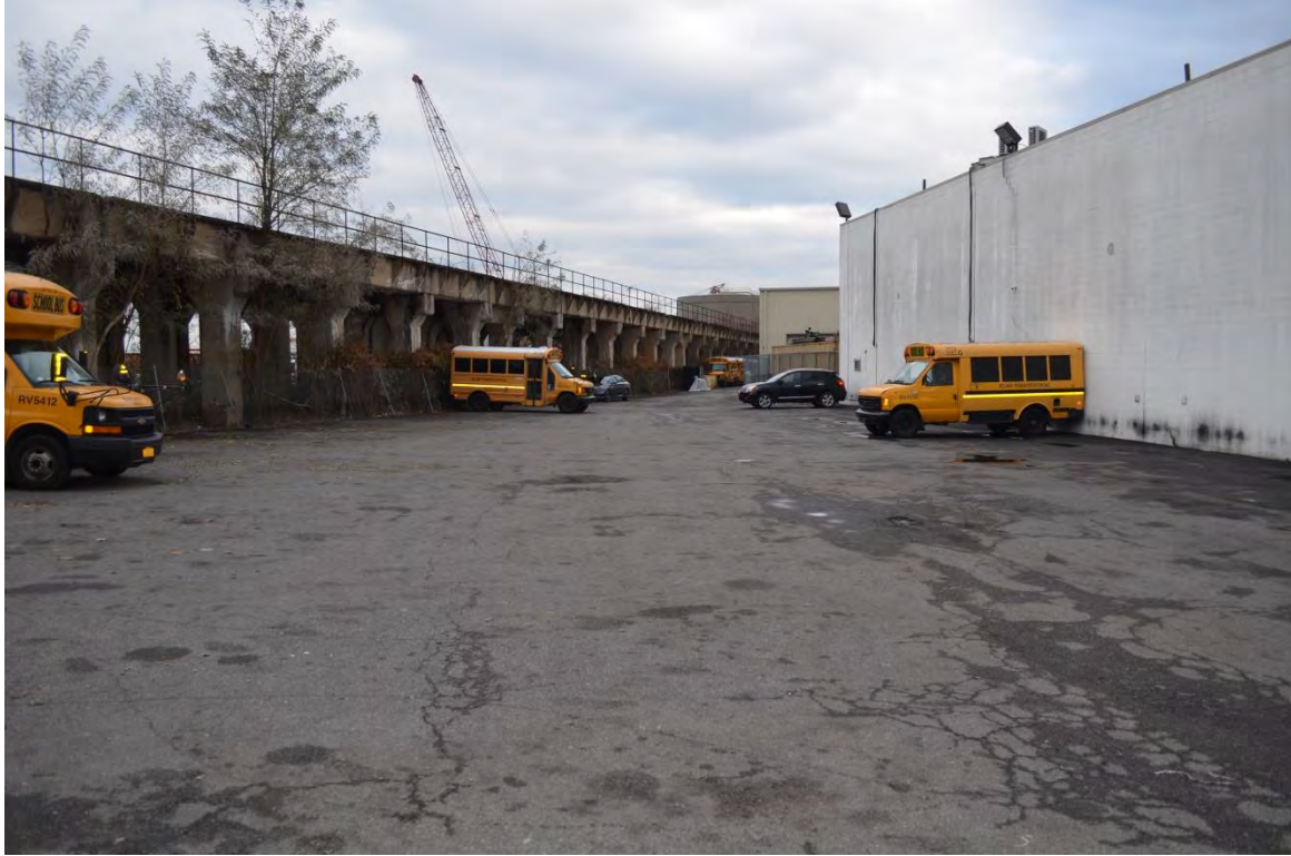
Photograph 27. Section 4, the viaduct near its crossing of Richmond Terrace. View looking northeast.
