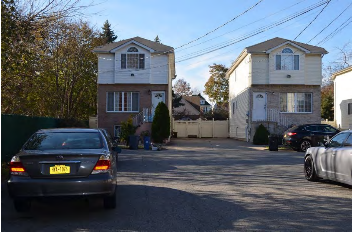
Photograph 5.31. Beamer Court north of the ROW. 40 and 50 Beamer Court (Block 1188, Lots 254 and 252). View looking west.
