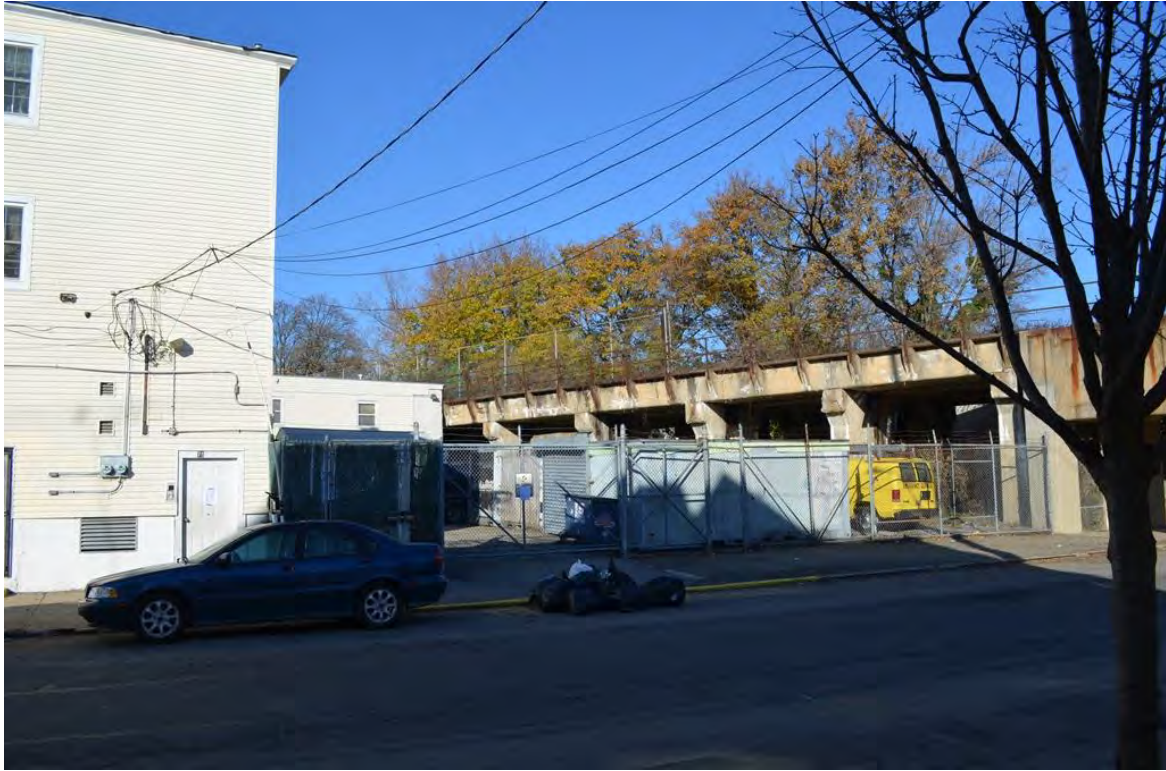
Photograph 4.25. Faber Street south of the viaduct. 78 Faber Street (Block 1076, Lot 1). View looking northwest.
