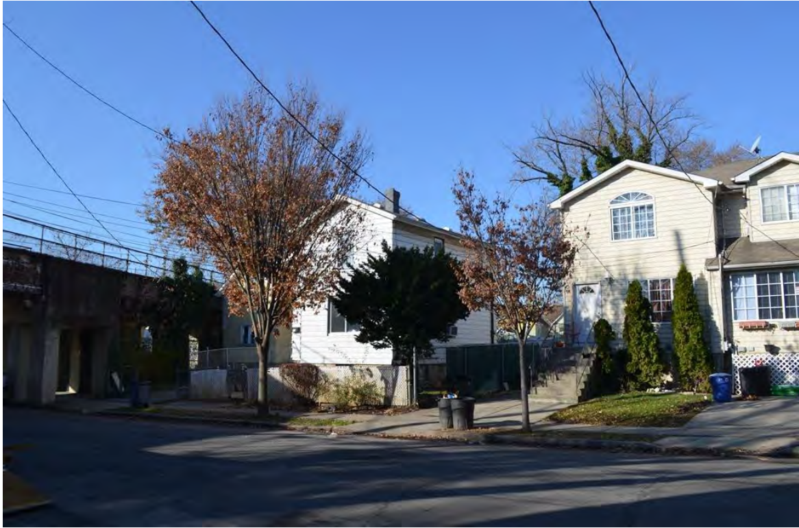
Photograph 4.27. Faber Street north of the viaduct. 56, 60, and 64 Faber Street (Block 1076, Lots 58, 56, and 53). View looking southwest.
