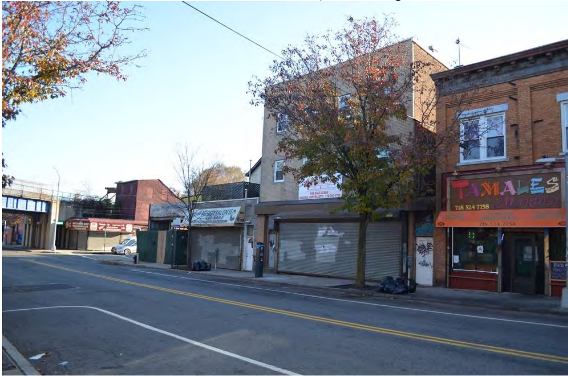
Photograph 4.16. Port Richmond Avenue south of the viaduct. From left: 81, 91, 93, 97, and 99 Port Richmond Avenue (Block 1004, Lot 1, 7, 10, and 11). View looking northeast.
