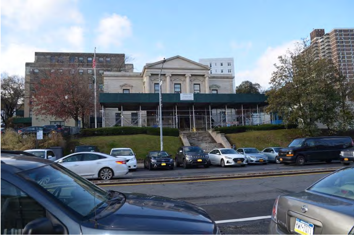
Photograph 1.11. Staten Island Family Courthouse, 100 Richmond Terrace. View looking west.
