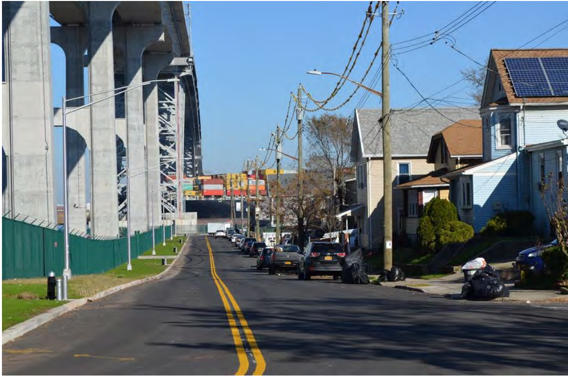
Photograph 5.10. Newark Avenue north of the ROW with the Bayonne Bridge approach on the left. From right: 81, 73, 67, and 65 Newark Avenue (Block 1123, Lots 3, 4, 7, and 10). View looking northeast.
