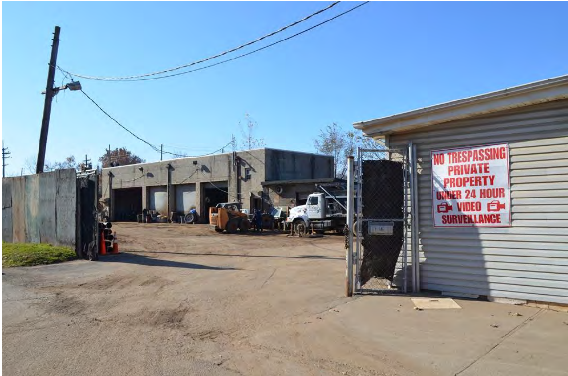
Photograph 5.11. Winant Street north of the ROW. 40 La Salle Street at the edge of APE (Block 1155, Lot 85). View looking southwest.
