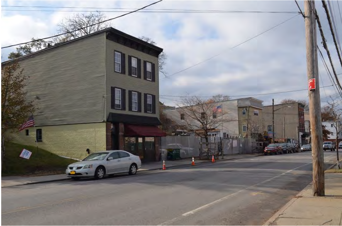
Photograph 2.9. Richmond Terrace, between Lafayette and Clinton Avenues, view looking southwest.
