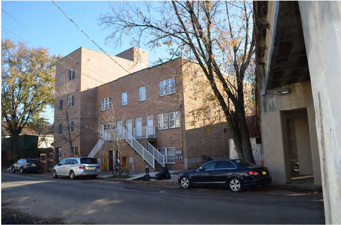
Photograph 4.20. Maple Avenue north of the viaduct. From right: 47-51 Maple Avenue (Block 1073, Lots 23 and 24). View looking northeast.
