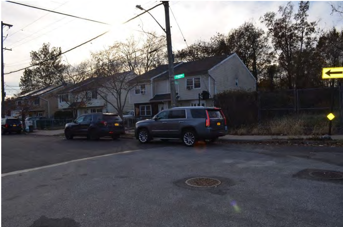
Photograph 6.8. Grandview Avenue and Roxbury Street south of the ROW. From right: 310, 312, 314, and 316 Grandview Avenue (Block 1261, Lots 93, 94, 96, and 98). View looking southeast.
