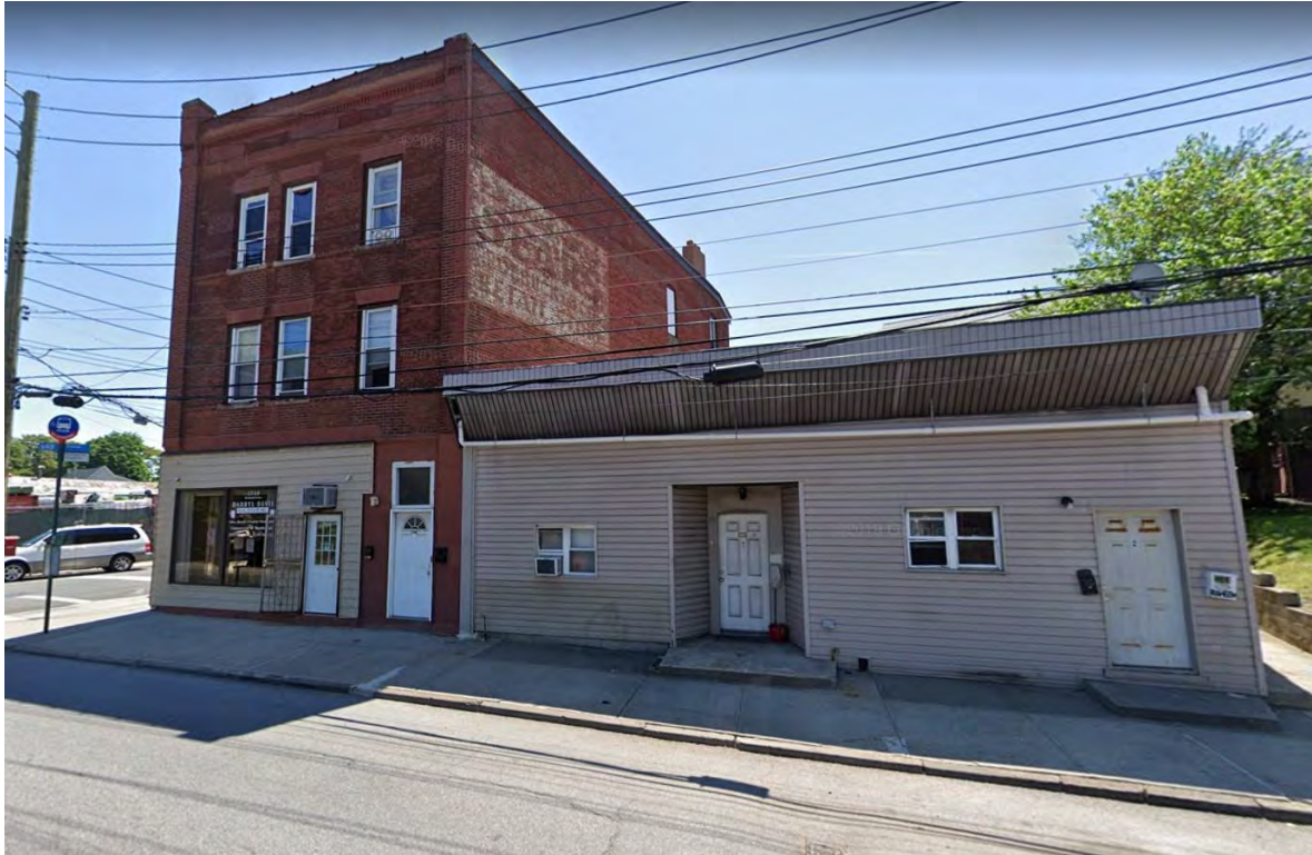
Photograph 4.3. 1740 Richmond Terrace. View looking southeast.
